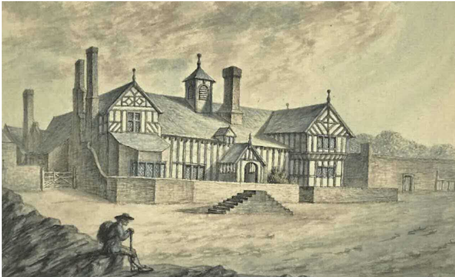
Fig 3. Churton Hall, 1793, drawn by J. Ingleby (Image: National Library of Wales). Note the wall next to the lateral chimney of which remnants remain; the outbuildings to the rear, which were rebuilt in the early 19 th century. Also note the central chimney stack, the eaves line which is roughly parallel to the timber framing wall plate, the walled garden to the west and entrance. At this point the Georgian side door hasn't been built. There are mounting steps for a carriage to the front of the wall of the hall.
