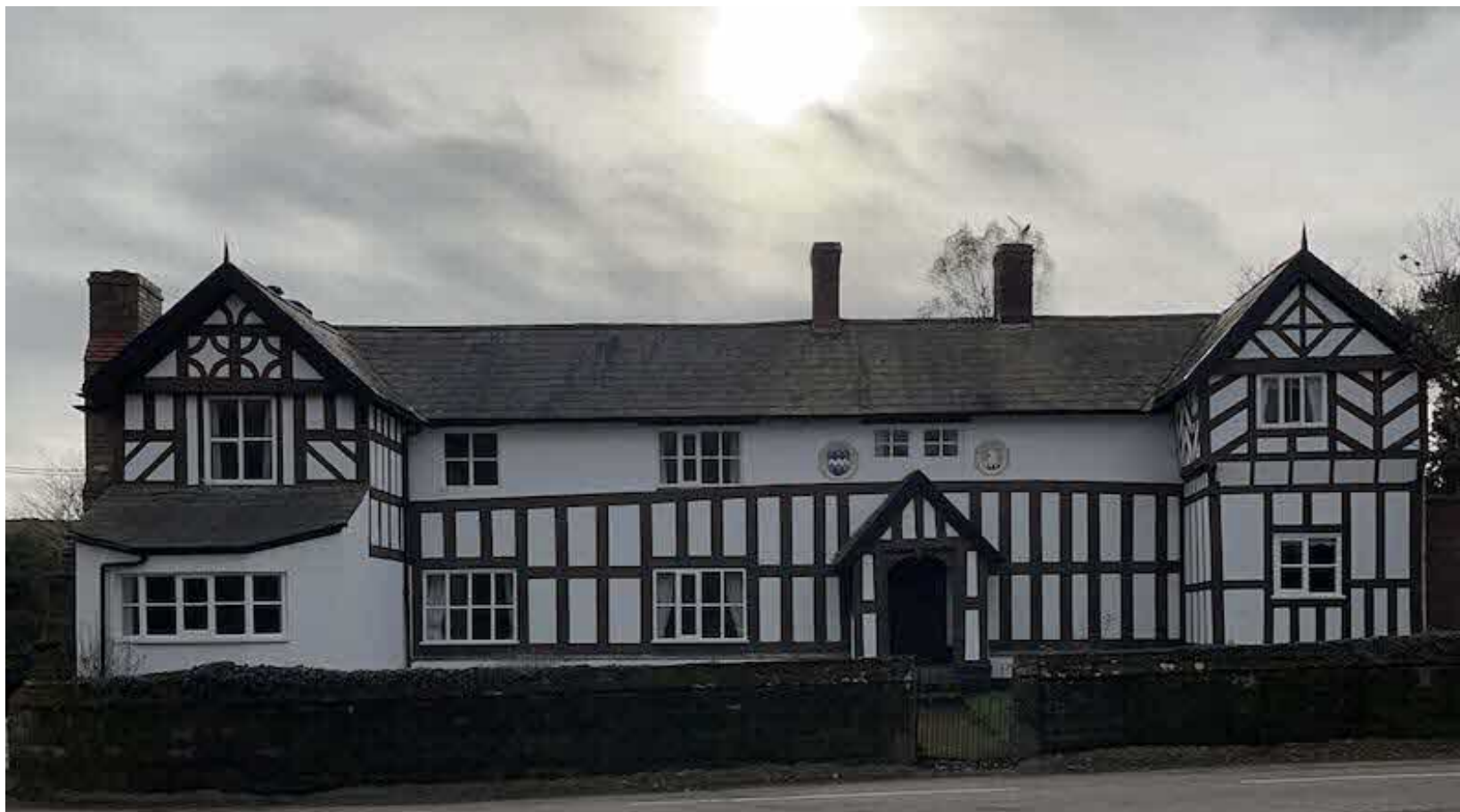
Fig 4. Churton Hall, 2023. Note the raising of the roof, probably undertaken in the 19 th century, with 19 th century casement windows; the smaller windows above the porch that replaced a dormer window; the off centre first floor window to the west wing; the central chimney stack is a late 19 th or early 20 th century addition the right chimney has been altered. The lateral chimney stack to the east gable has been truncated. The north west projecting gable perhaps retains some 19 th century vernacular revival chevrons to the first floor.
