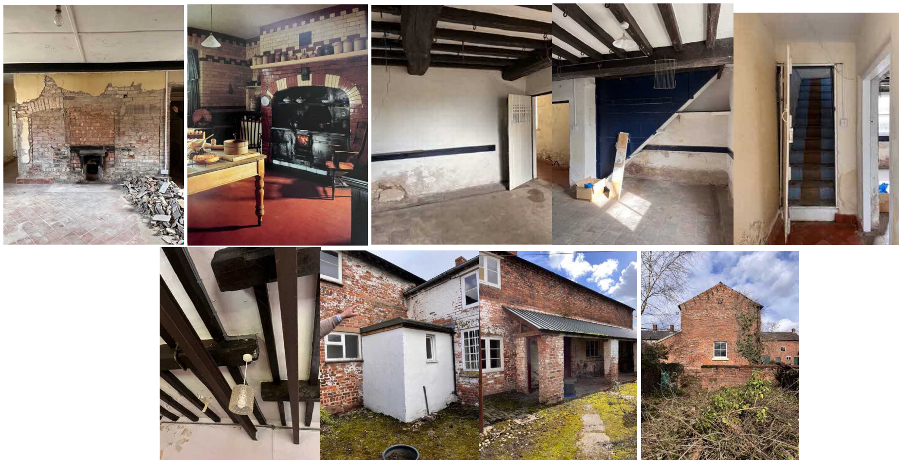
Fig 22. Features of the Victorian wing including from top left to right: the former kitchen range area – the second image is from ‘The Victorian Society Book of the Victorian House’, image 3 and 4 show the meat room and the later staircase to be removed, which will reinstate the room proportions. Bottom left to right; evidence of a missing wall to be reinstated, the flat roofed modern WC behind main house; the functional veranda to be removed – former dairy area; and the south facing gable.
