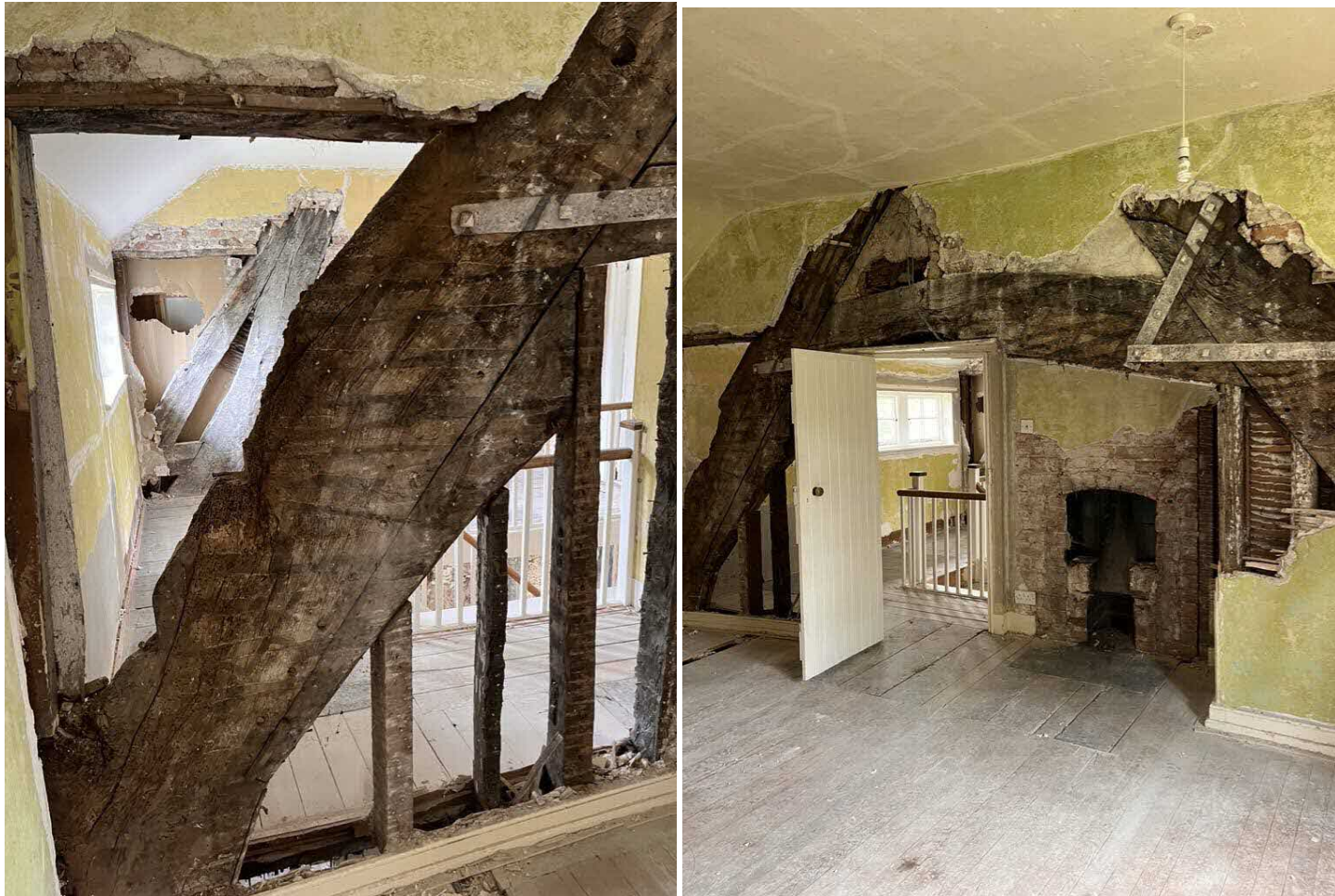
Fig 11. The raised cruck to the west of the existing hallway. The 'upper' face of the truss faces west, into the bedroom, suggesting that this faced the most important end of the house.
