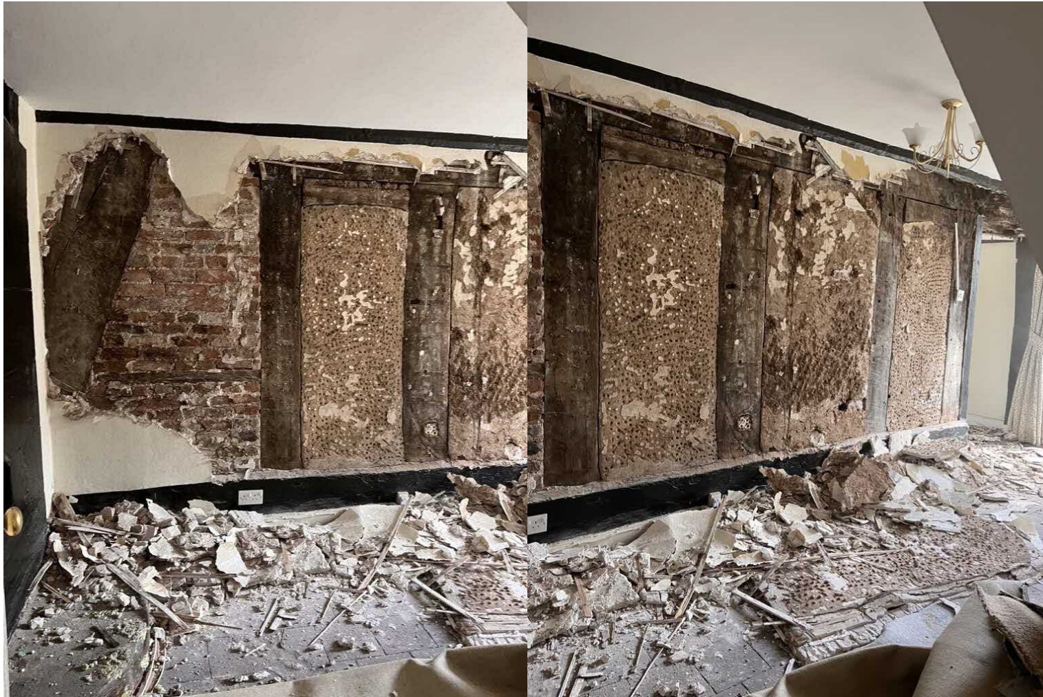
Fig 7. The assumed screens partition within the cross passage. Note the cruck to the left of the first photograph.
