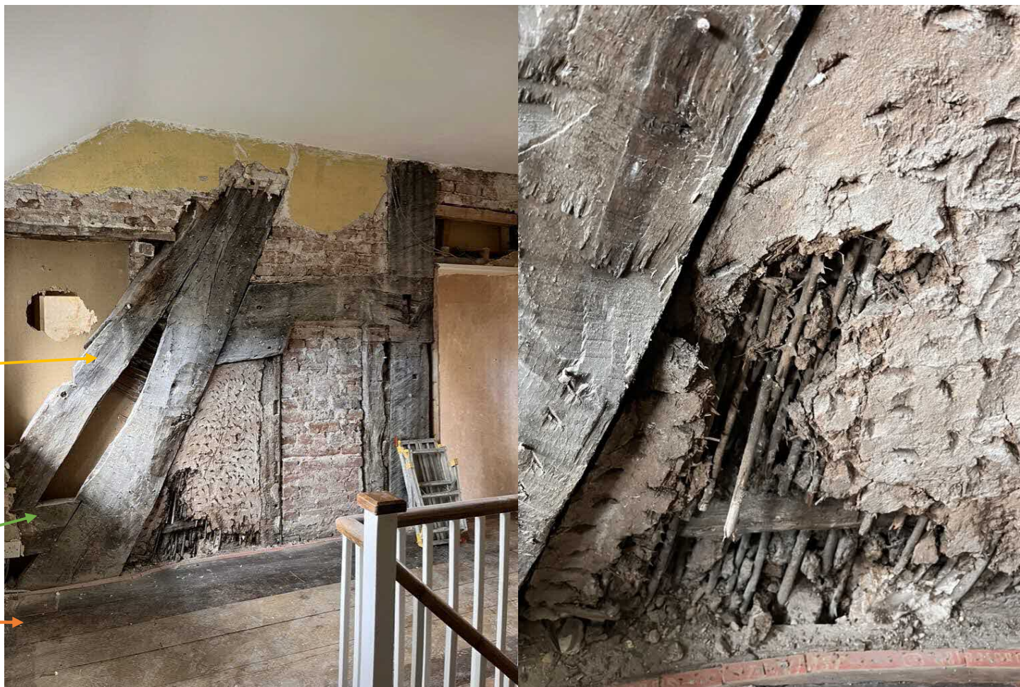
Fig 9. The cruck to first floor above the screens partition showing wattle and daub and later brick infill. Note the packing piece (arrowed yellow) and the spur (arrowed green). The tie beam (arrowed orange) at floorboard level appears original to the truss.
