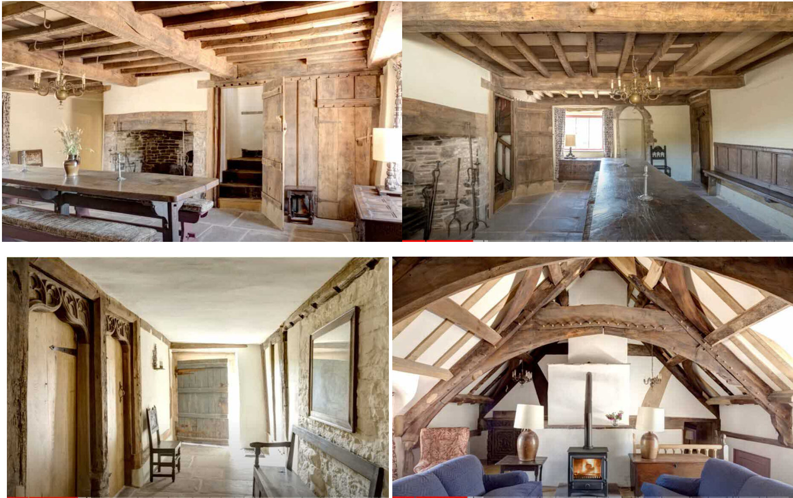
Fig 16: Llyn Celyn, Monmouthshire (Grade I) restored by the Landmark Trust. Note the 17 th century fireplace and stairs, and restored timber finishes (top photos); the cross passage (bottom left); the cruck frame with arched brace (bottom right)
