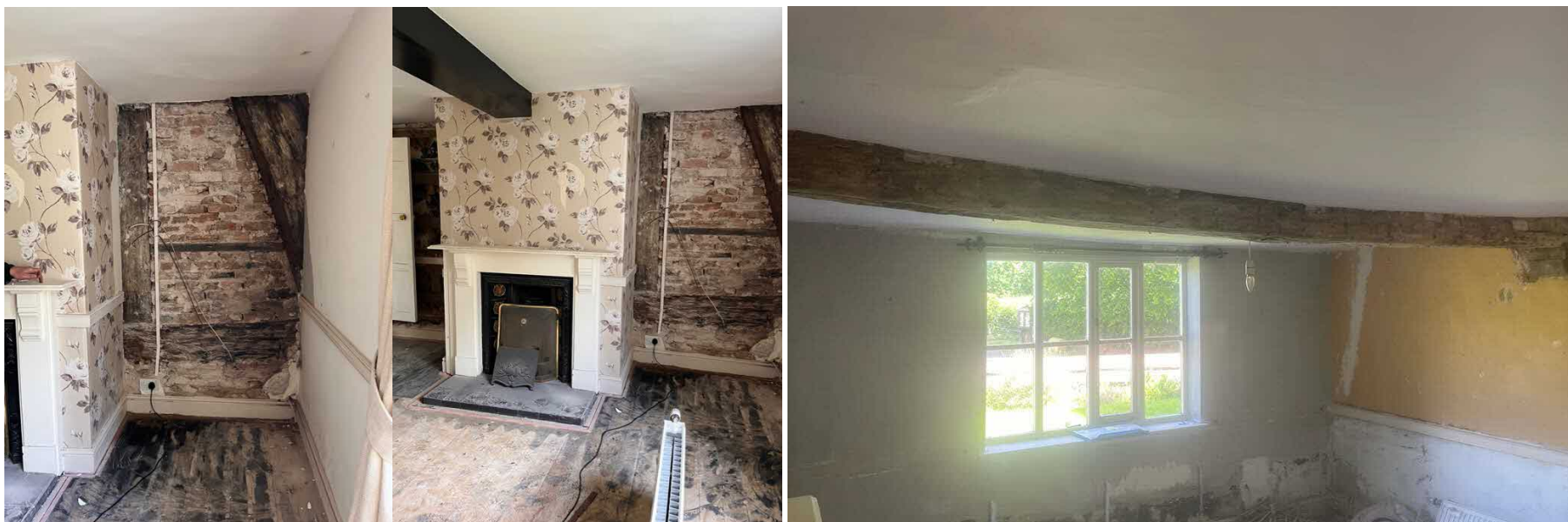
Fig 8. The other side of the screen passage inserted next to an early 20 th century fireplace. The floorboards were probably installed at the same time, or later. The sandstone cellar is underneath this floor. A stop chamfered beam is encased in plaster and painted black gloss. This has now been uncovered. It has been raised and is resting on a corbel that may indicate the location of the division wall between pantry and buttery.
