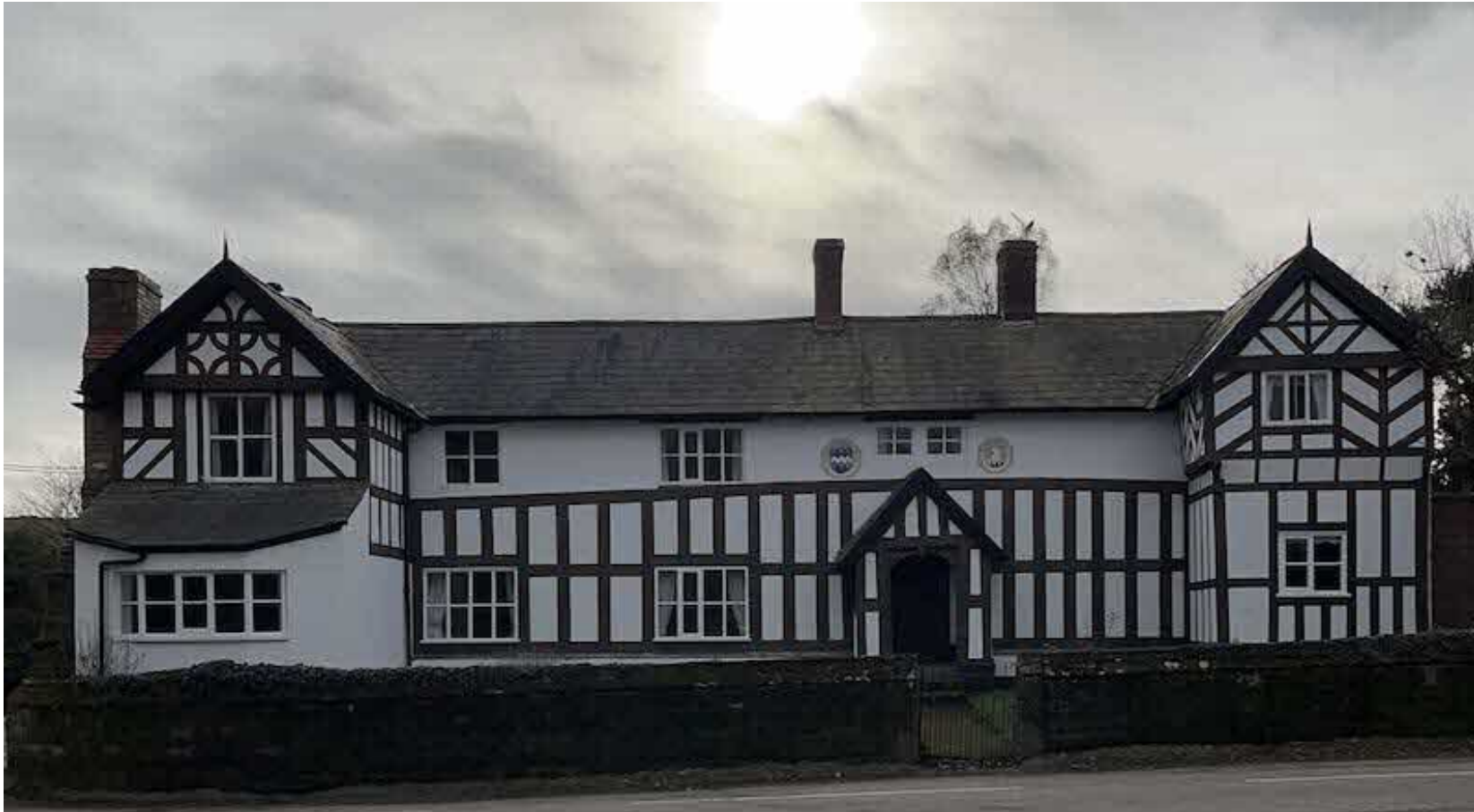
Fig 4. Churton Hall, 2023. Note the raising of the roof, probably undertaken in the 19 th century, with 19 th century casement windows; the smaller windows above the porch that replaced a dormer window; the off centre first floor window to the west wing; the central chimney stack is a late 19 th or early 20 th century addition the right chimney has been altered. The lateral chimney stack to the east gable has been truncated. The north west projecting gable perhaps retains some 19 th century vernacular revival chevrons to the first floor.
