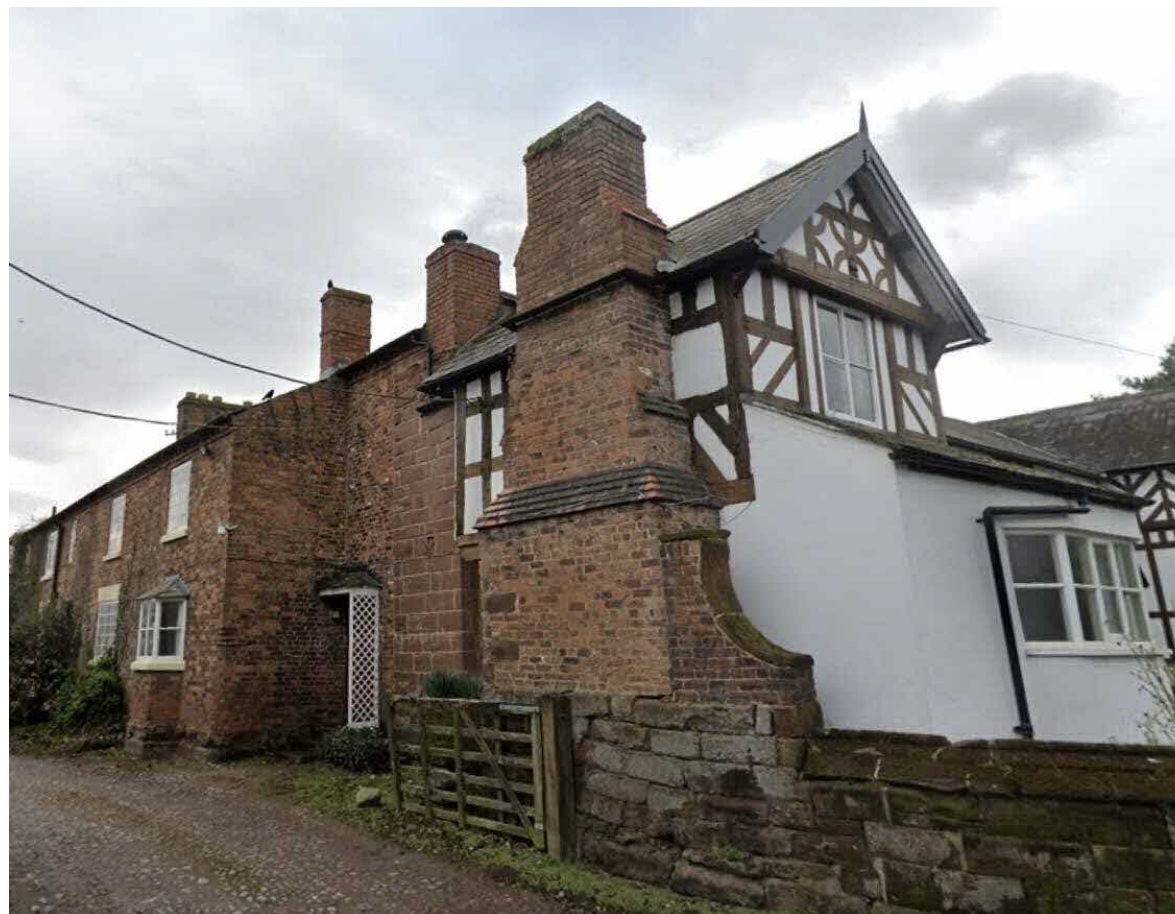
Fig 6. The east wing of the house, with a service wing to the rear. Note how this has changed since the 1793 drawing. There is a two storey wing, which appears to be one build and is early 19 th century. This has metal small paned windows. There is a side entrance from the farmyard, which suggests that this became the primary entrance. It is a six panel raised and fielded Georgian front door, probably early 19 th century. Internally there is a door of the same age leading to the early 19 th century wing. The bay window to the left of the latticed entrance door is later 19 th century, this room was the farm office.
