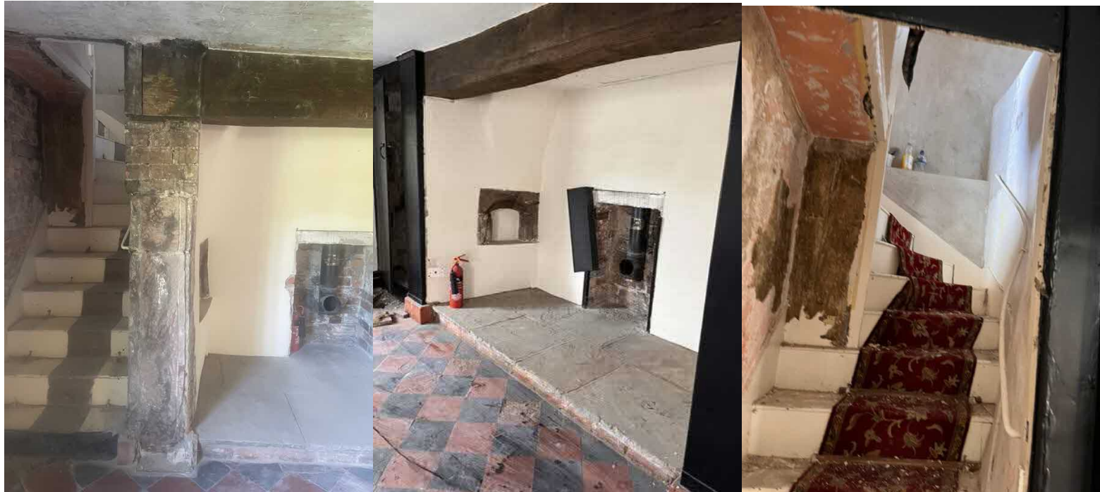
Fig 13. The altered inglenook on the east wall; the bread oven; stairs to the side of the fireplace leading up to two bedrooms. The tiles were probably added in the 19 th century on an earth floor.
