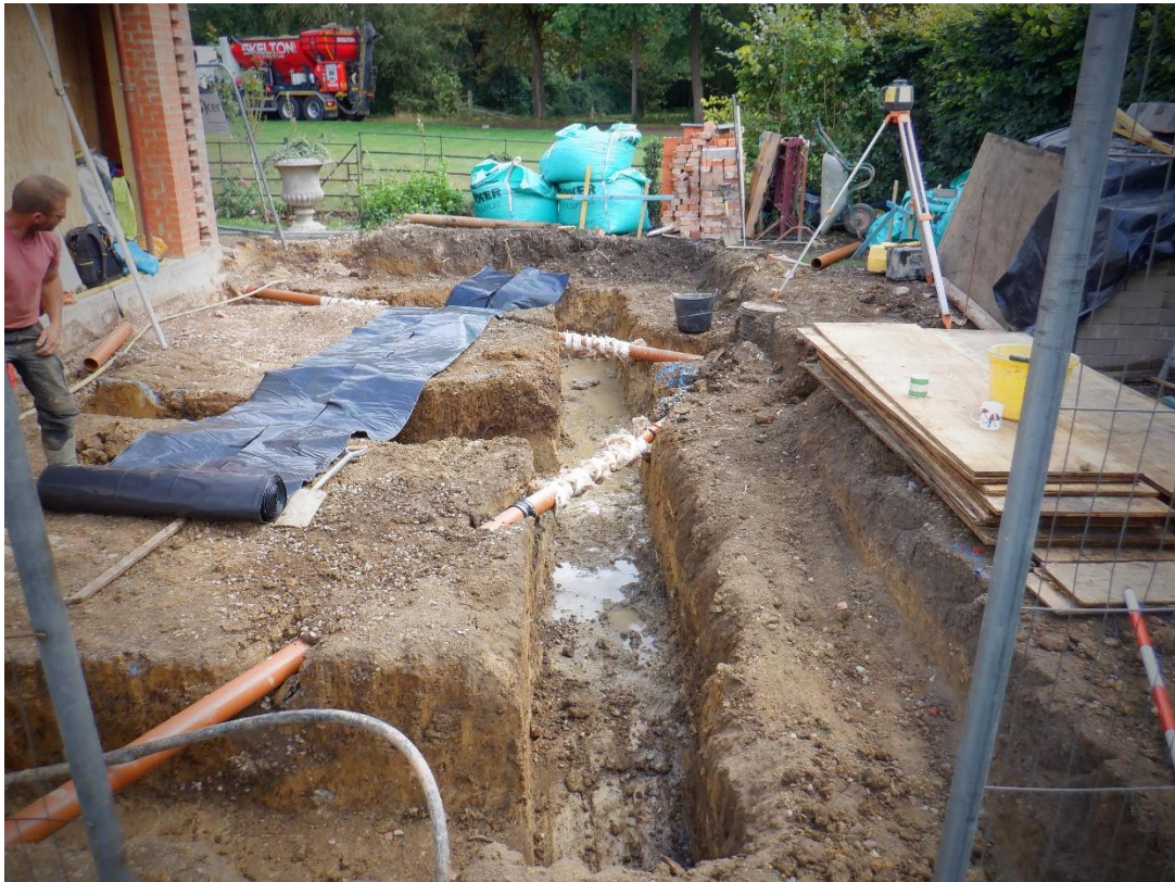
Plate 6. Foundation trenches (looking East)
