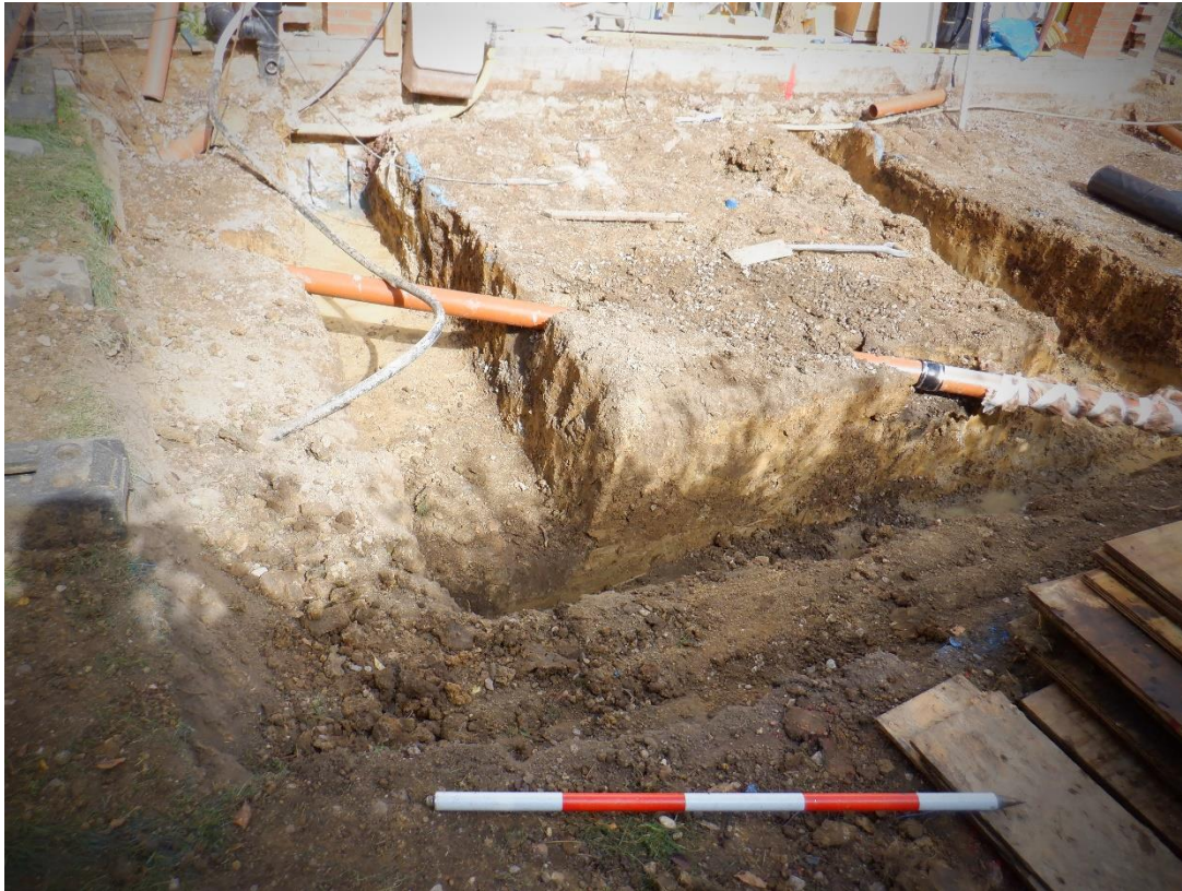
Plate 5. Foundation trenches (looking NE)
