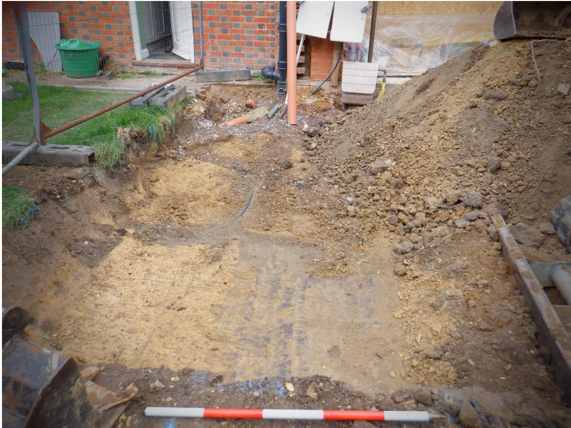
Plate 3. Ground reduction (looking NNE)
