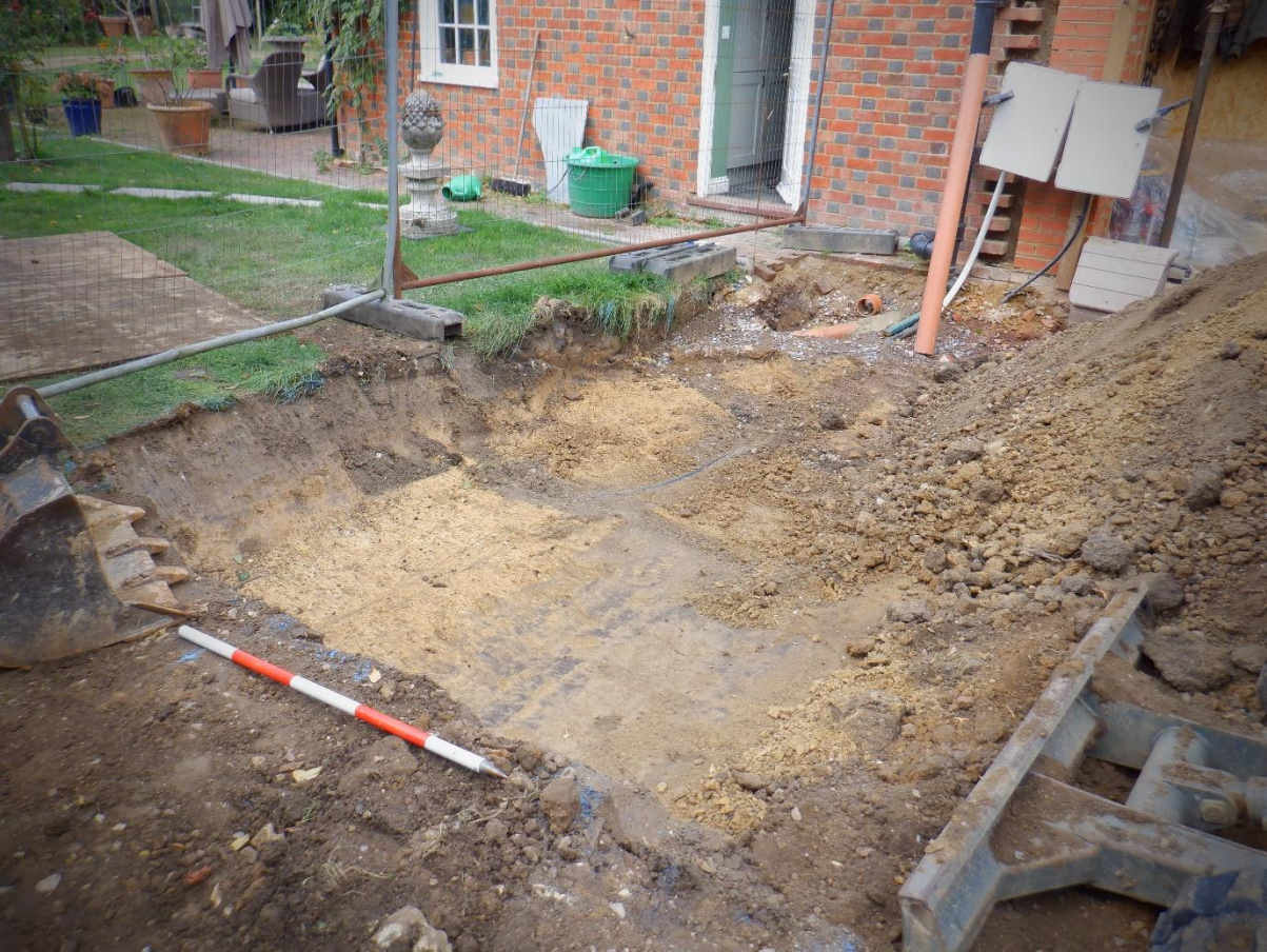
Plate 1. Setting out and starting ground reduction (looking North)
