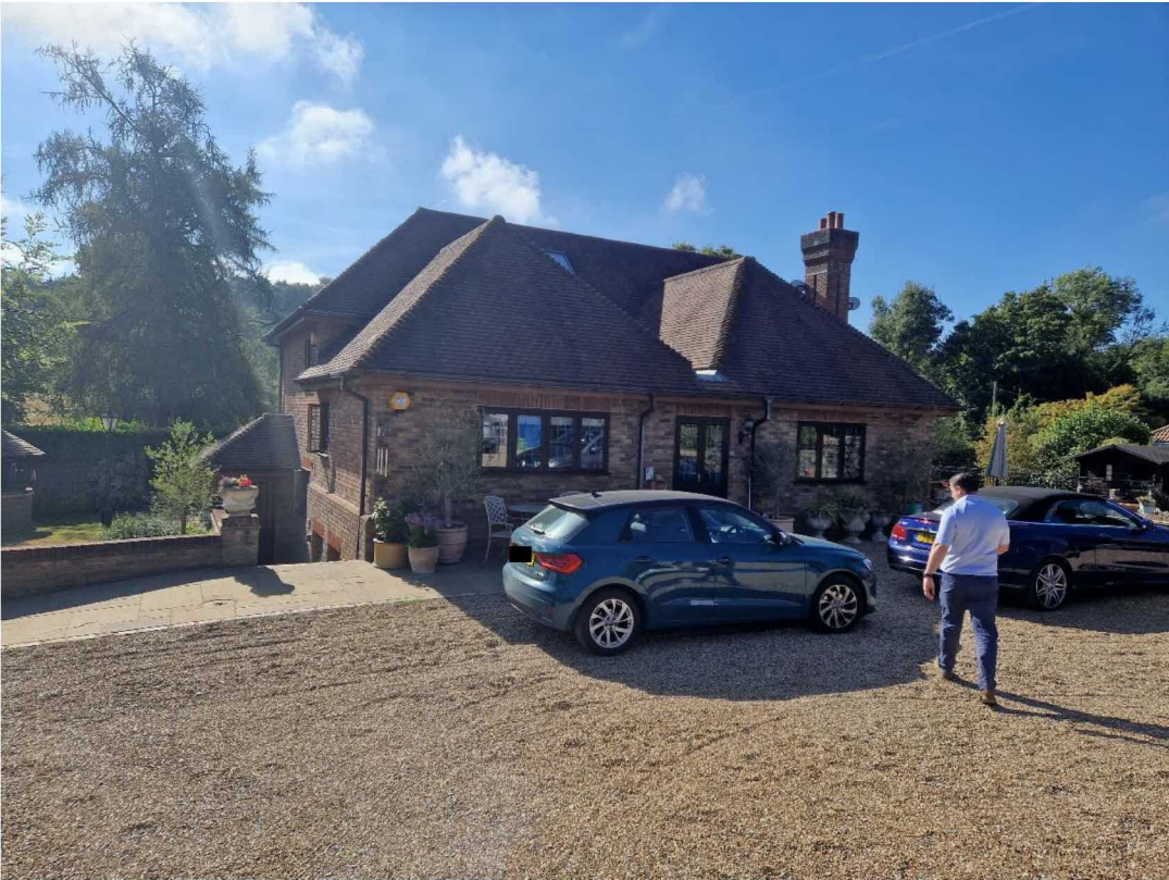
Rear View of the Main House
