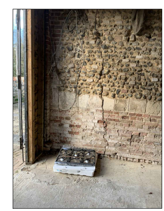
CRACKING LOCATION 1
