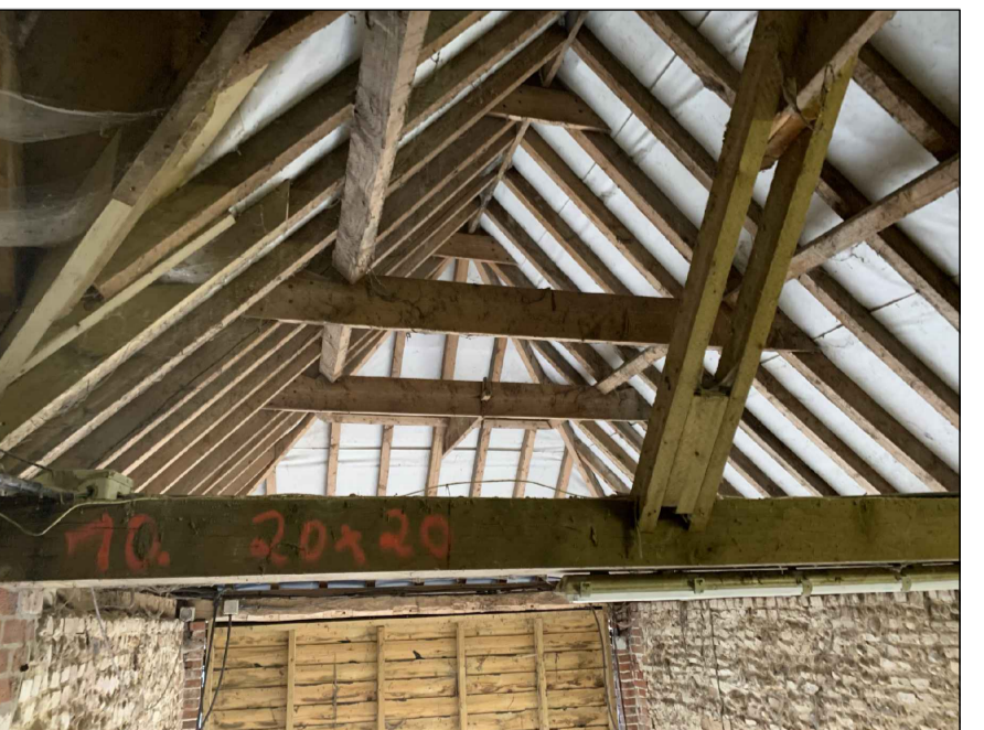
AREA WHERE FEATURE TRUSS IS TO BE INSTALLED
