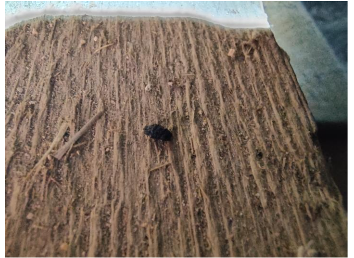
Photo 8 Bat dropping on stairs of stables
