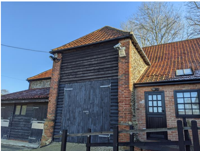
Photo 3 West elevation of the barn
