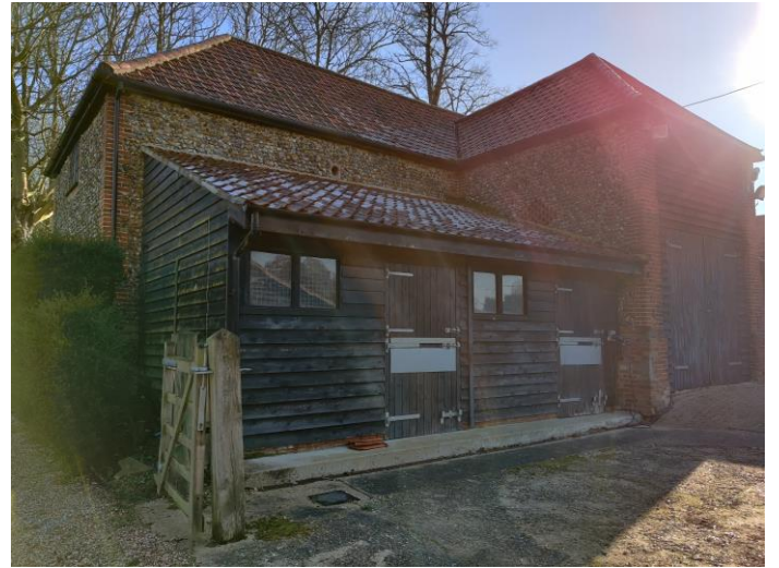
Photo 2 Northwest elevation of the barn with attached lean-to
