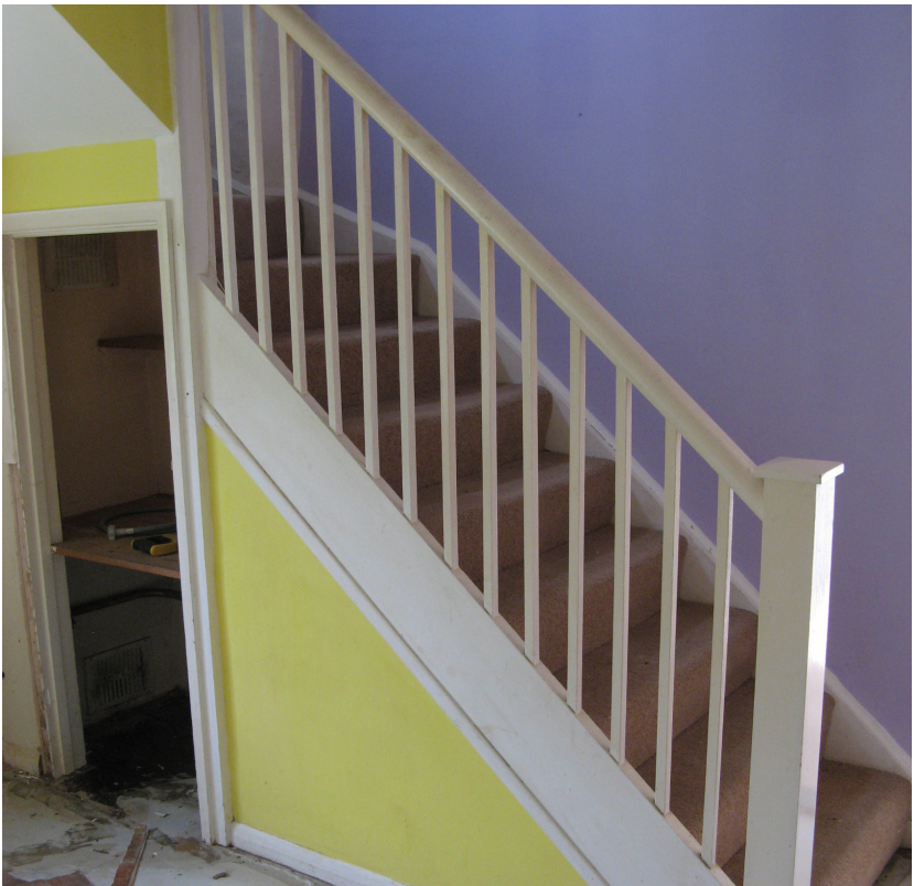
Staircase to be removed (No. 94).
