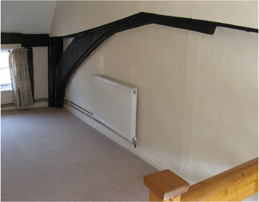
Arch braced tie beam and inserted first floor accross former open hall.
