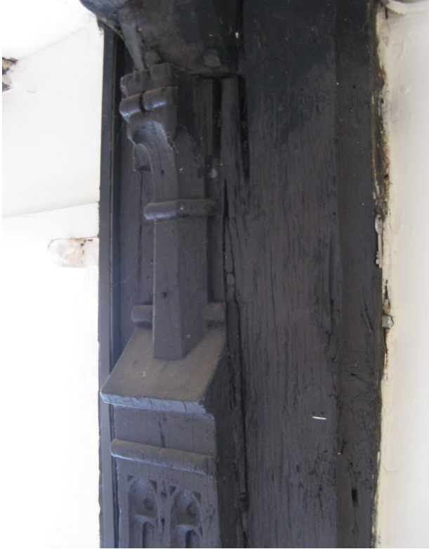
Carved principal post at ground storey. Later insertion of floor beam
