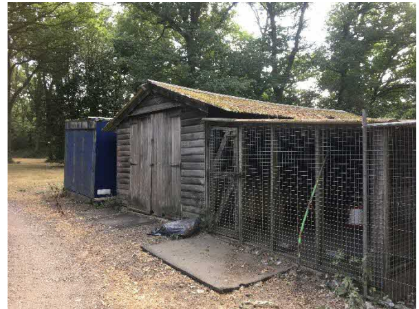
Photo 2: Eastern facades of storage container and kennel building
