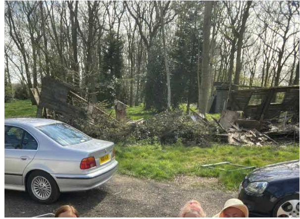
Photo 14: Northern façade of derelict building taken 2021 – very little bramble growth, partially covering central and western sections
