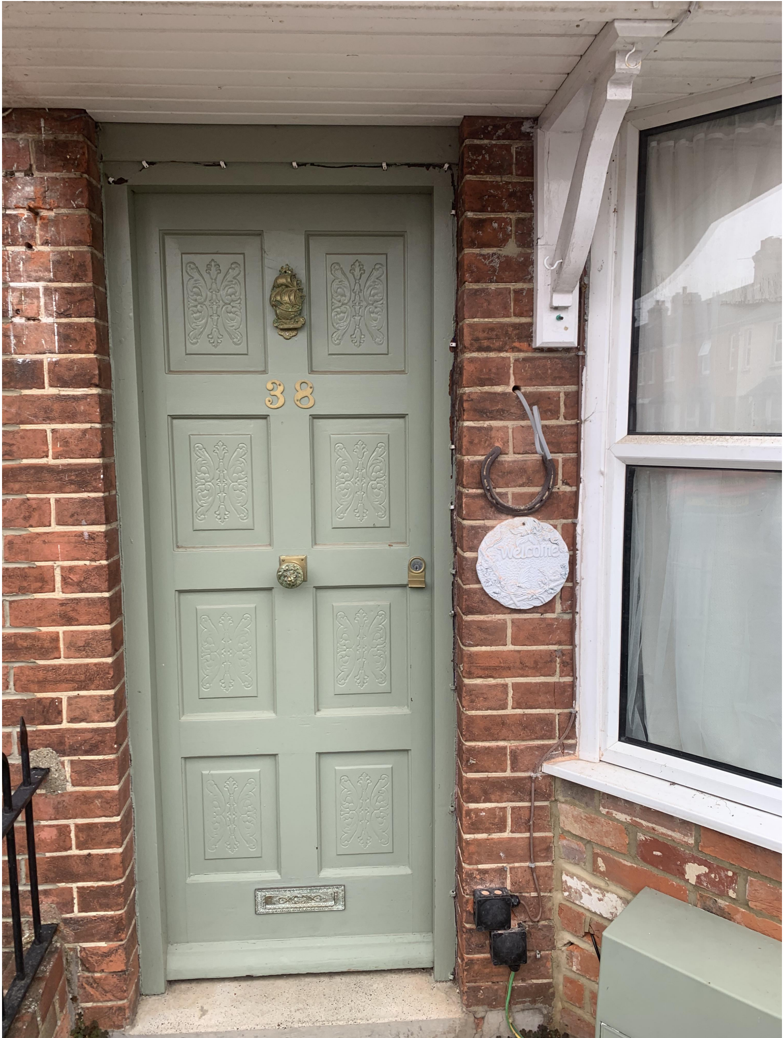
Existing Image - Door 02/10/2023
