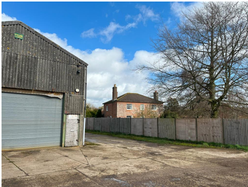
Figure 14: View of Rookery Farmhouse (grade II) from the application site
