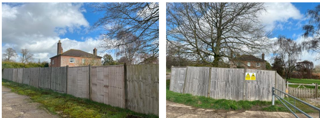
Figures 16 and 17: Views of Rookery Farmhouse (grade II) with a large fence in front
