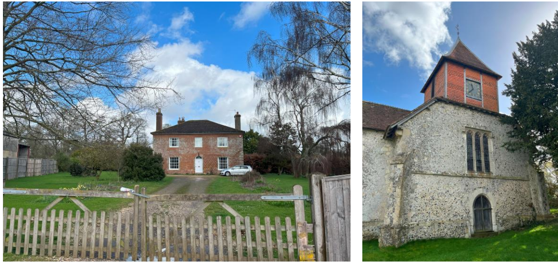
Figure 2: Grade II listed Rookery Farmhouse (left) and grade I listed Church (right)
