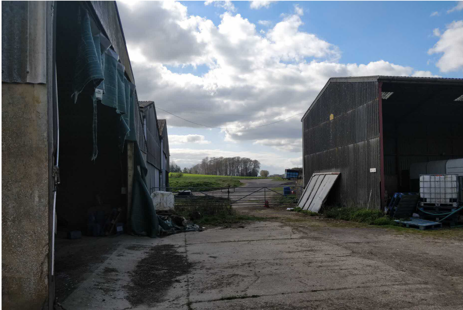
View looking west of existing agricultural buildings.
