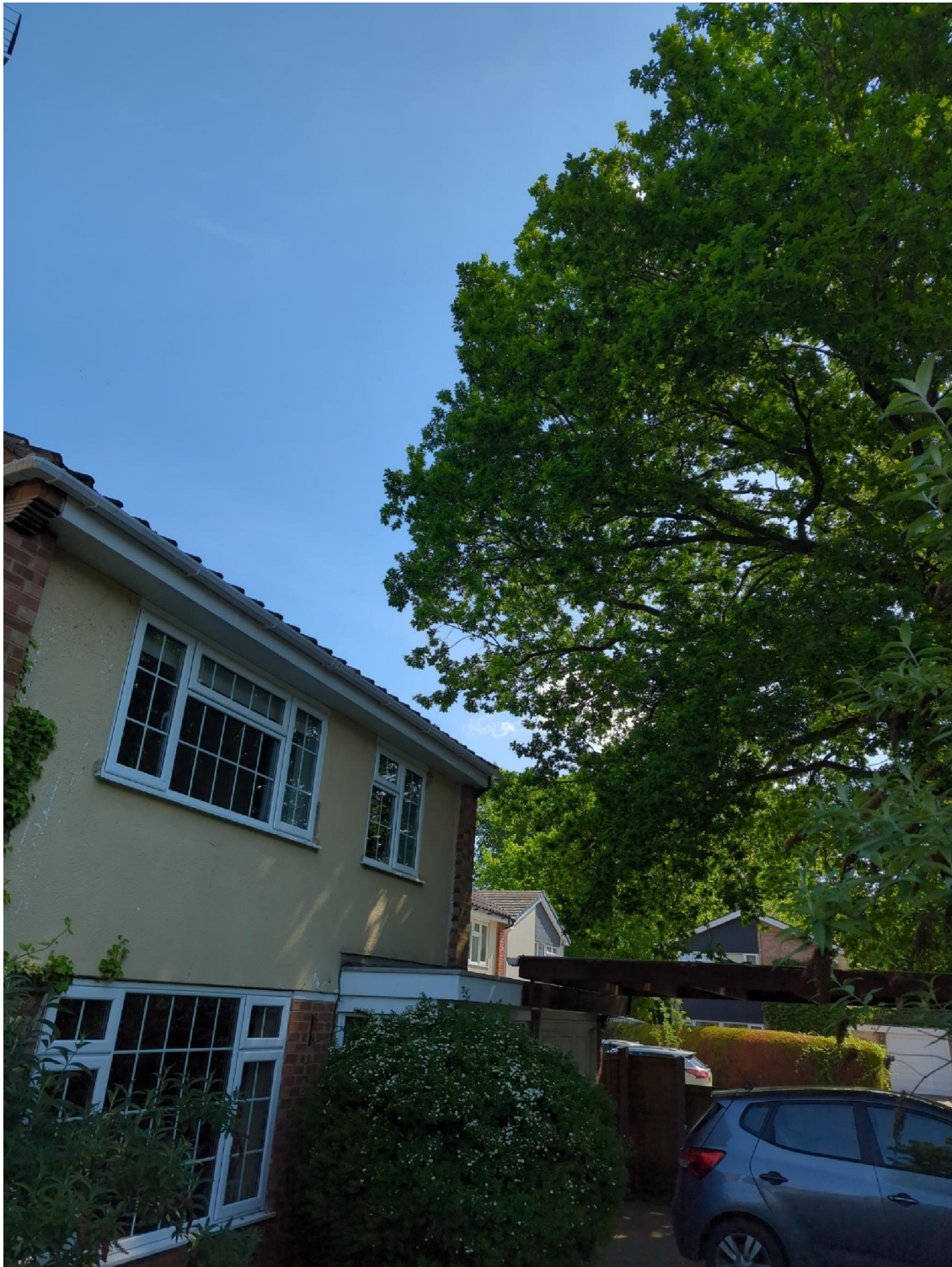
Photo 3 Closer view of tree and building.
