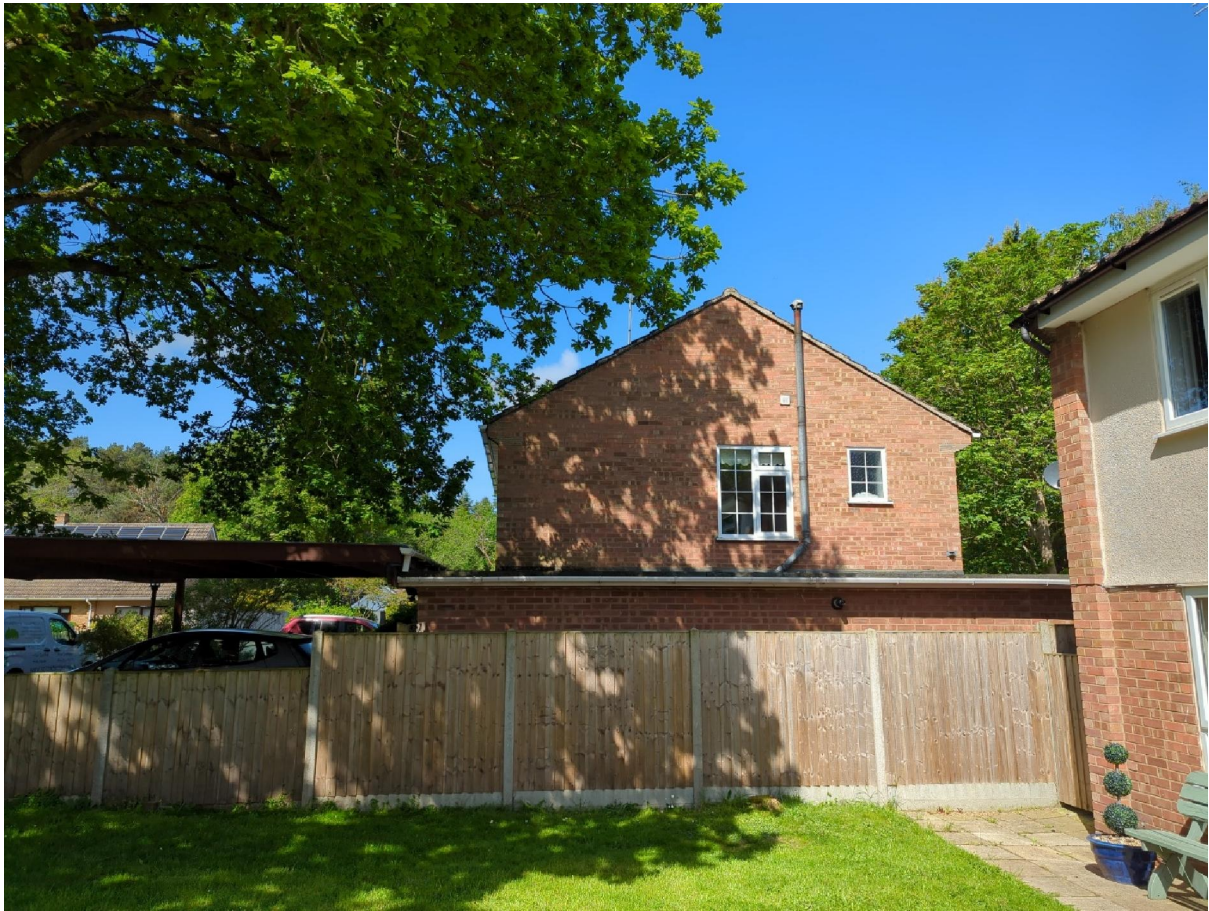
Photo 4 view from the South over area of proposed new structure.
