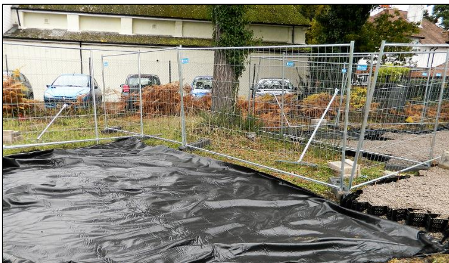
Figure 7. Photographs illustrating cellular confinement system used to form an above-ground no-dig driveway.
