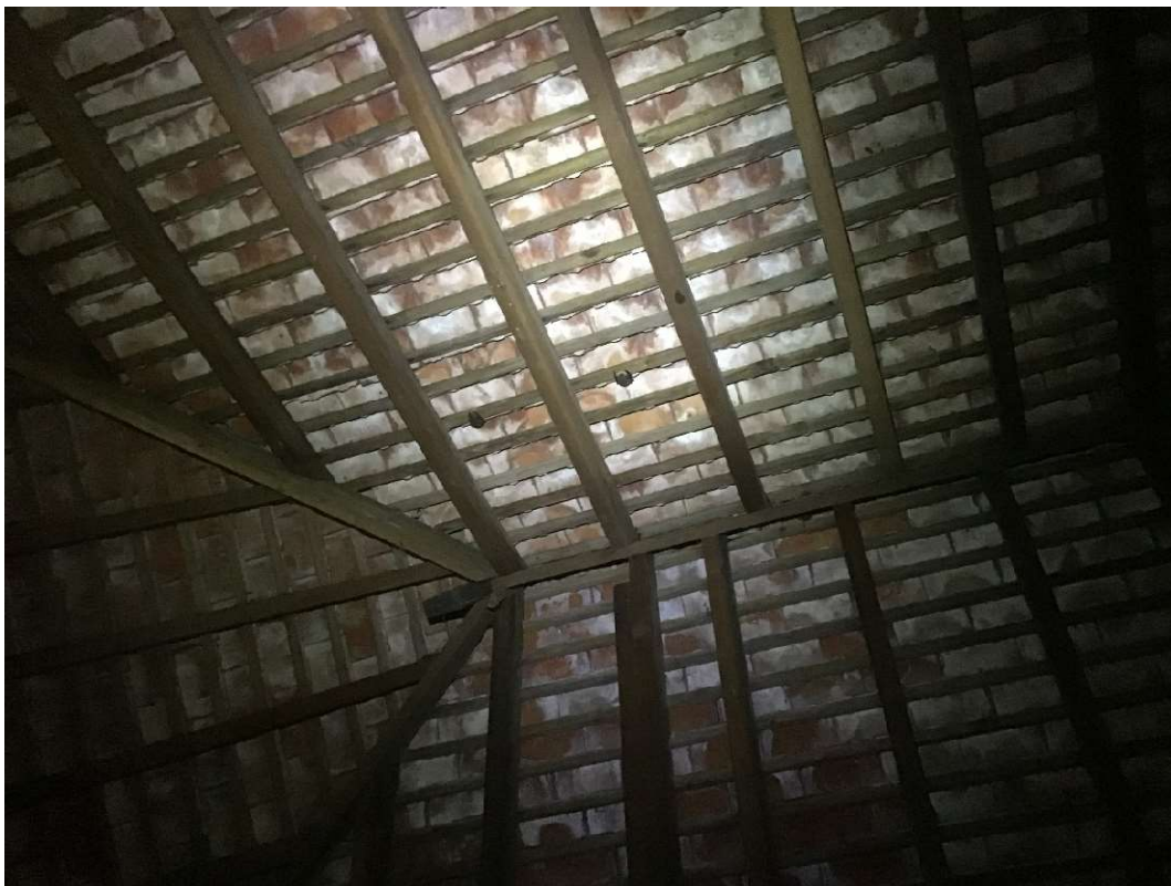
Figure 6. Loft with brown long-eared bats in situ .
