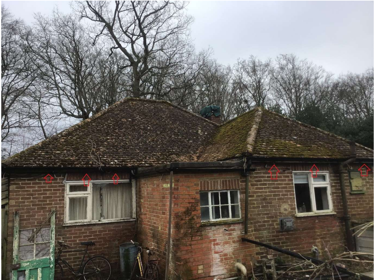
Figure 4. Northern elevations looking south. Red arrows indicate potential access points for roosting bats,
