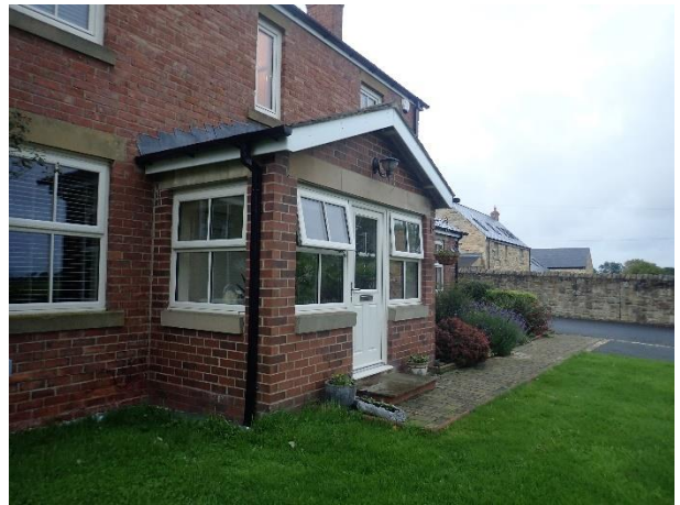
Mortar fillet missing in places
