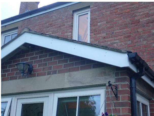
Mortar fillet missing in places
