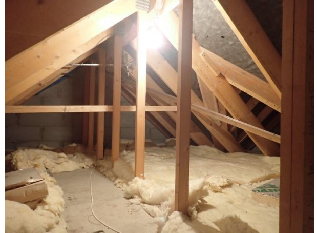
Main house loft space, evidence of cluster flies and occasional mouse dropping
