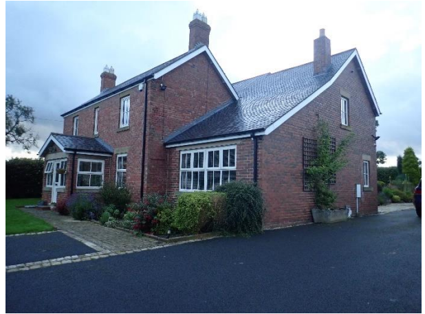
The north aspect from the northeast
