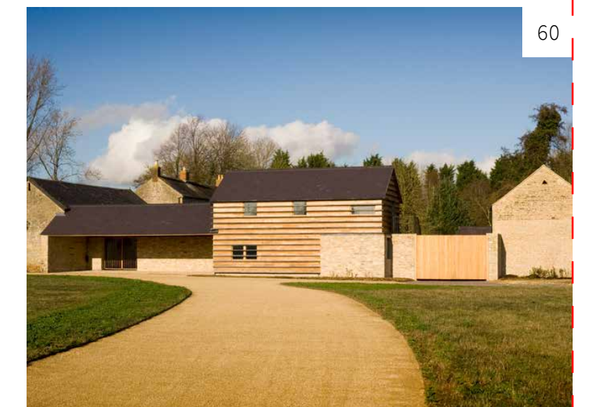
58-59 An archive and office have been inserted into the shell of a disused building on a working farm. Two new timber structures sit within the old walls with a new roof over-sailing each.
