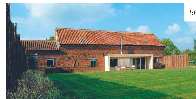
Images 57-60 57 This carefully designed new extension has used the walls and footprint of an old piggery. A new link has been made to the main barn.
