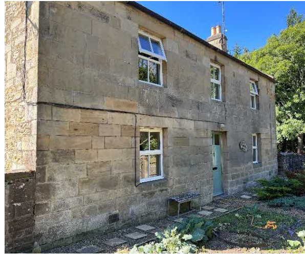
The 'modern' casement windows to the east elevation
