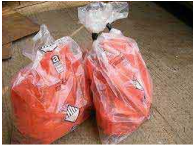
Typical double bagged asbestos waste
