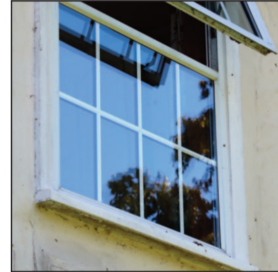
Glazing bars are sandwiched between glass.
