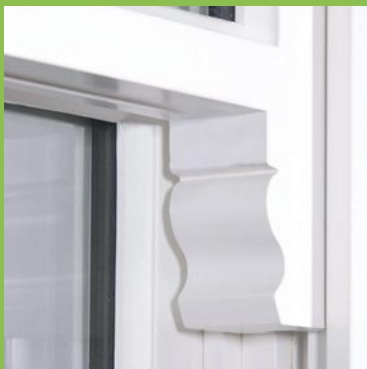
Horn detail to sash
