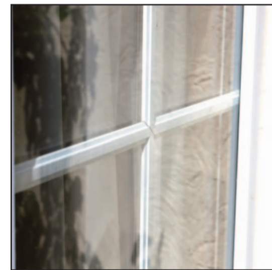
Glazing bars are sandwiched between glass.
