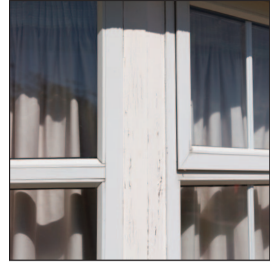
Aluminium windows construction within a timber bay frame.
