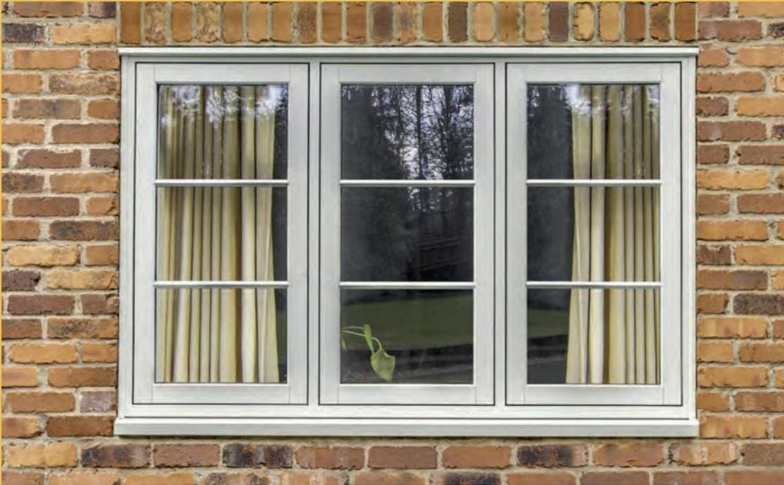
Flush casement window with Genus timber-style joints to frame and sashes
