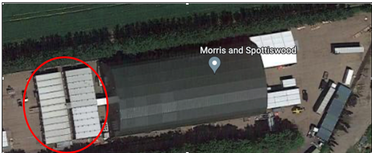
Position of Portable Production Offices as seen on aerial imaging – unit sizes 12m x 3m (26 in total) – source Google maps
