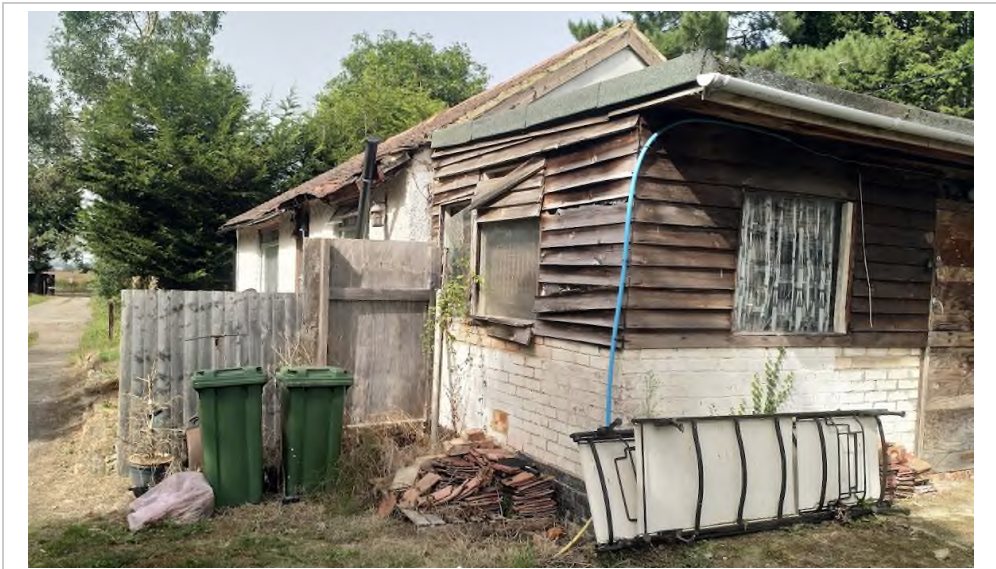
Image 4: The existing dwelling – Side Elevation. Retained under planning application 22/00281/FULL
