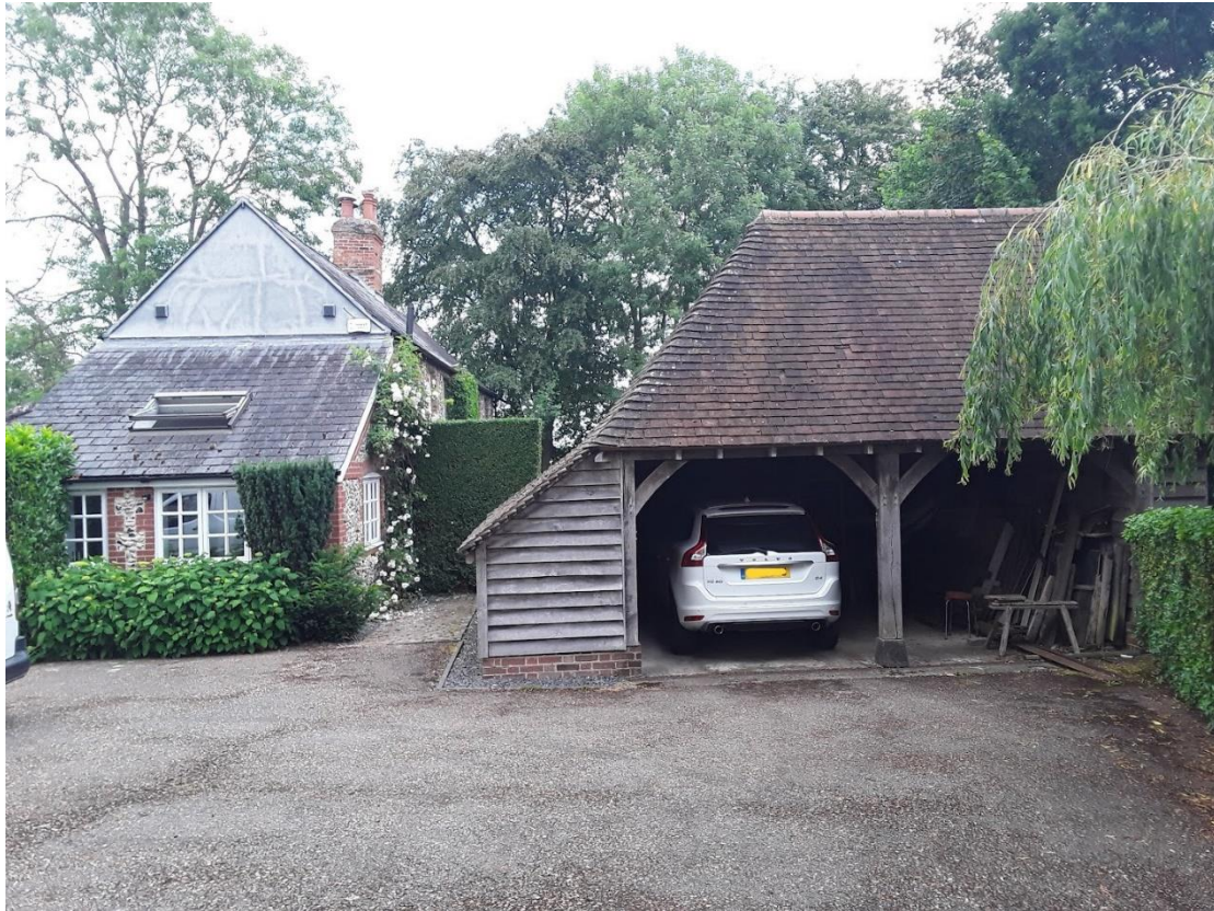
Figure 2 – Looking eastwards at the existing garage (to be demolished)
