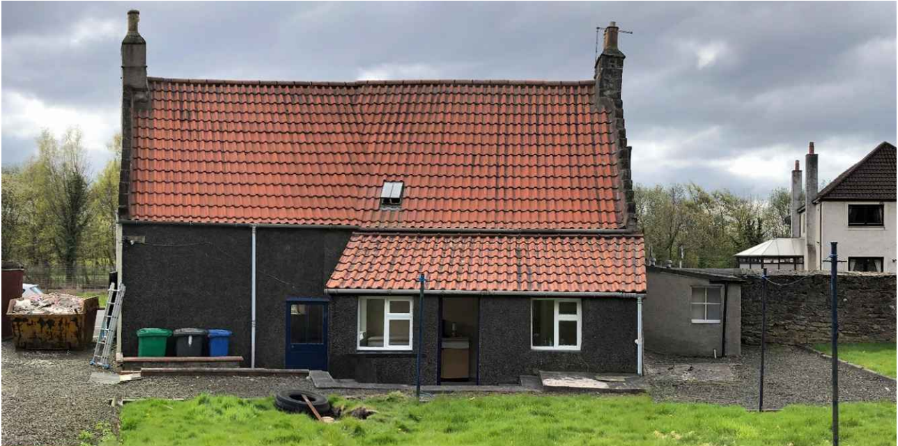
Figure 18: The north elevation of Westend Cottage showing 1980's roof, black harling, and uPVC windows in the Victorian kitchen extension. In the background is the development from 2000's that has a major impact on the visual amenity and historical setting of Westend Cottage.
