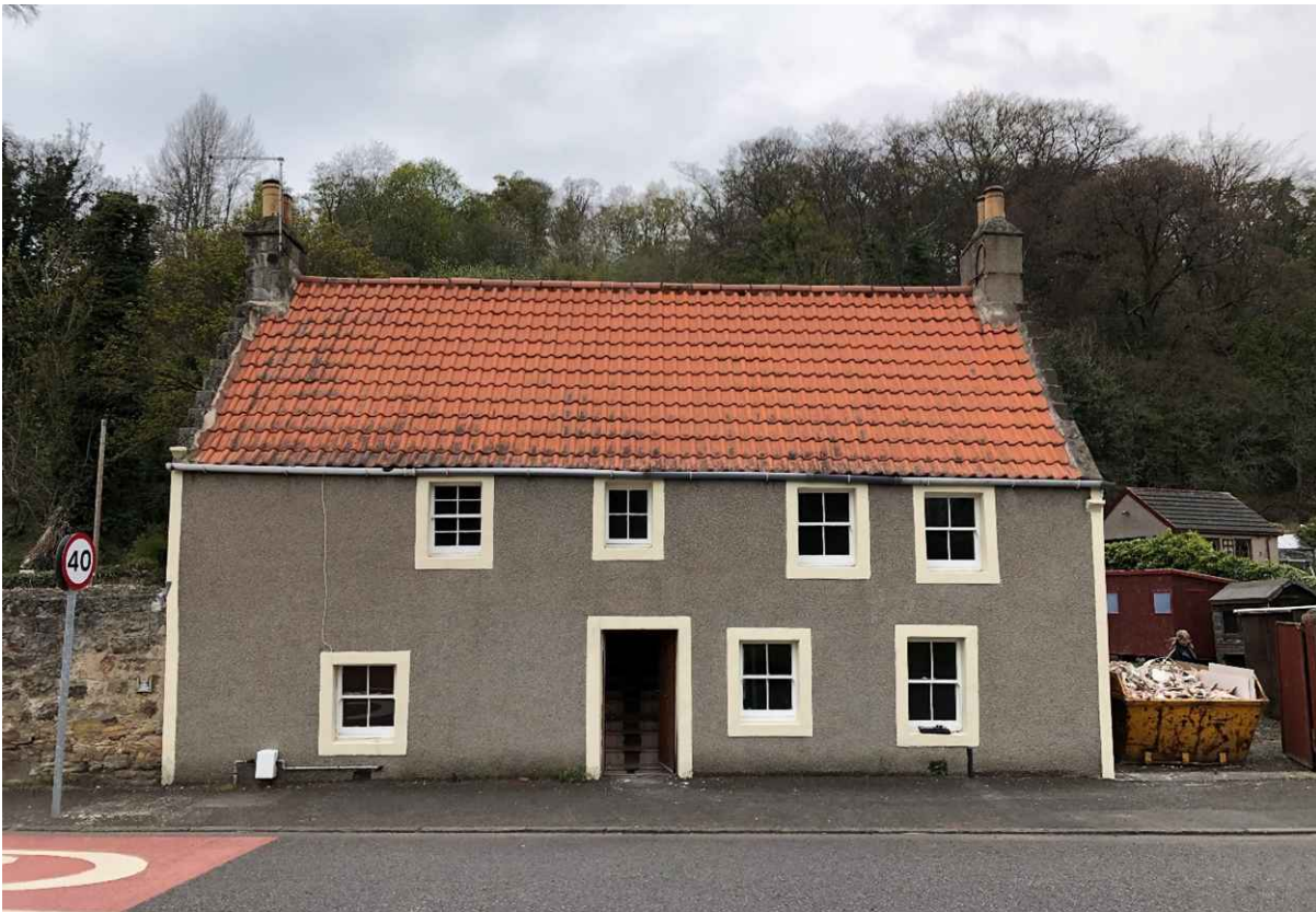
Figure 12: South elevation showing change in pavement height
