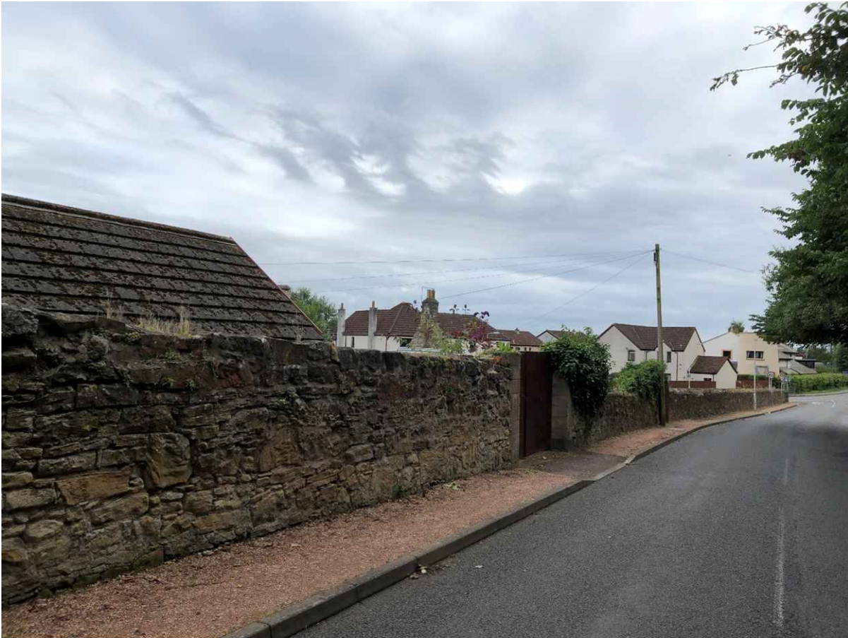
Figure 9: View south from Low Causeway Road. Note the boundary wall height provides good screening into the property. Google Maps shows a different view which is achieved by a camera set at 2.5m high which gives a false perspective of visual amenity and overlook into the property.
