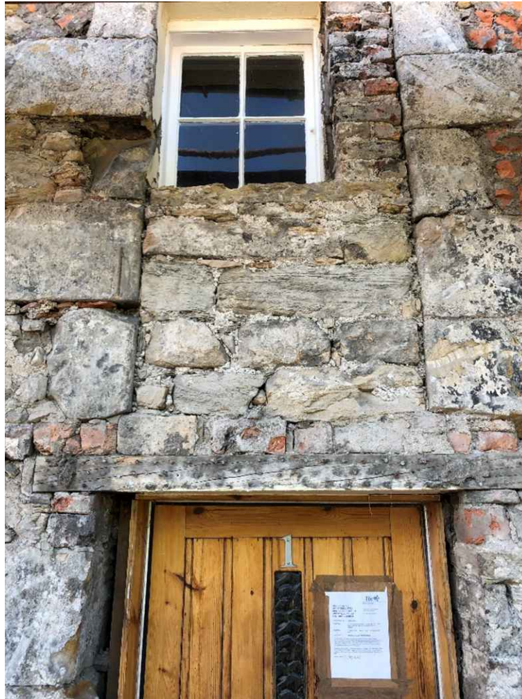
Quoined returns at the front door that show the building was once two distinct buildings. The quoins run down to grade
