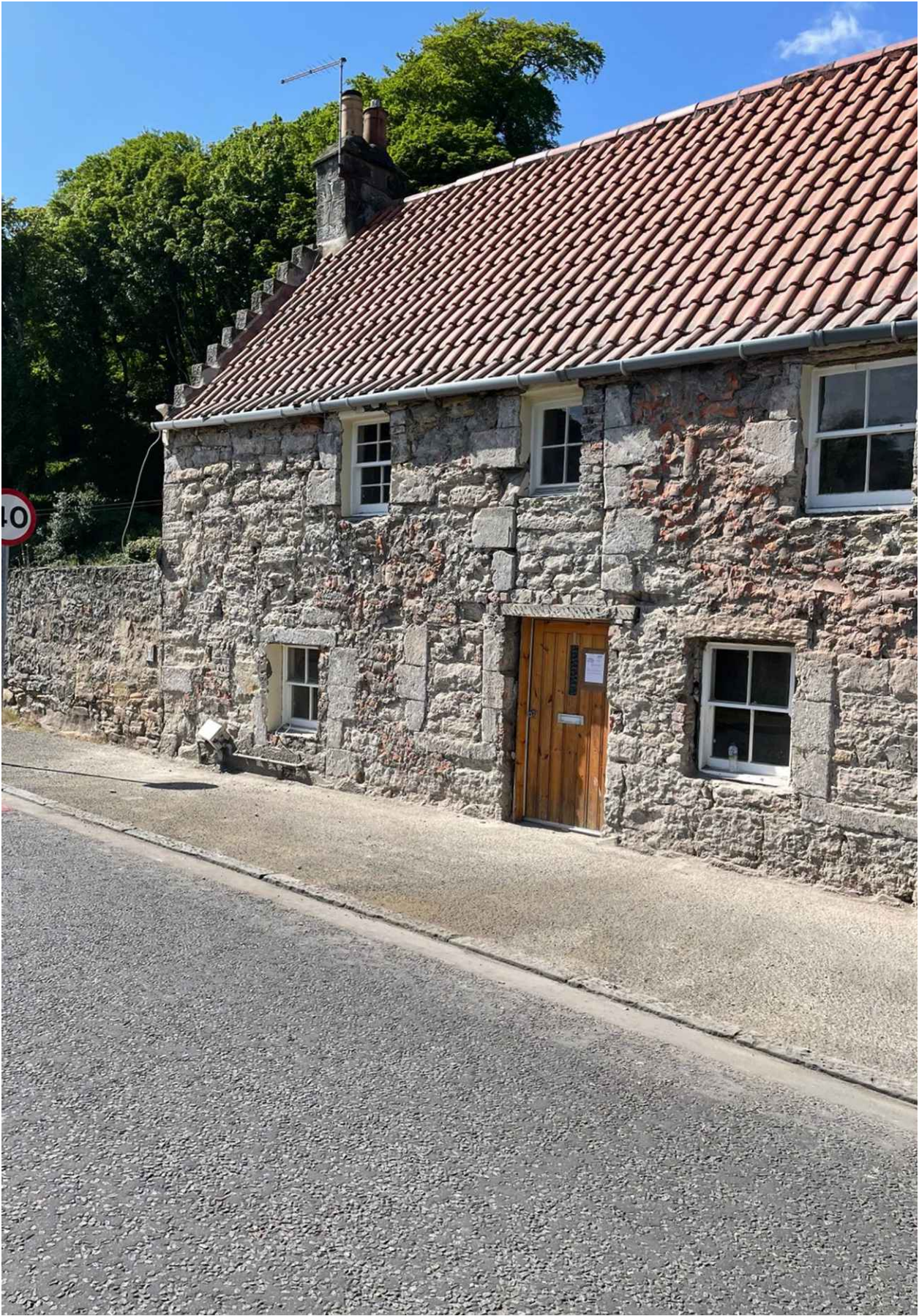
Figure 17: Original windows filled in with sandstone, either side of the front door. Quoins above the entry showing the infilled pend that once separated the two buildings. Brick and cement infill to fill in gaps in the wall for the cement render applied in the 1960's
