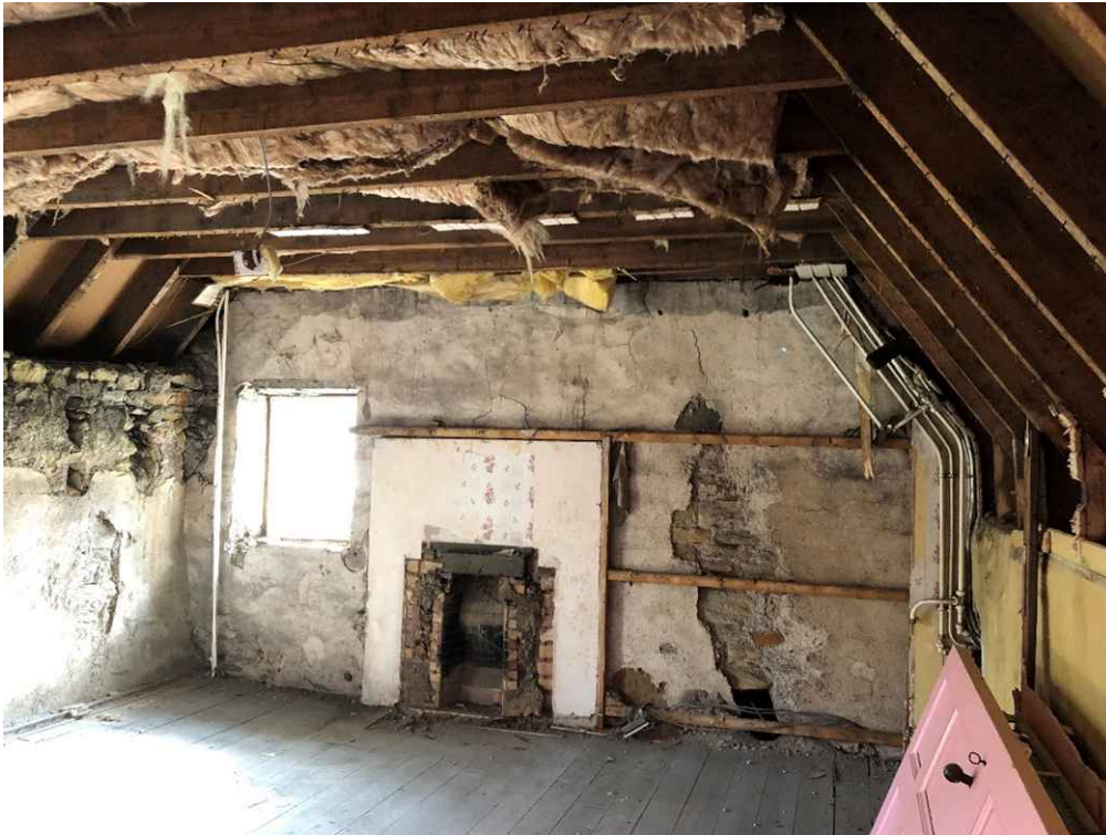
1 st Floor west bedroom. Stripping back to original wall construction. Note holes in the wall on the south side and at floor level from the exposed ground floor flue.
