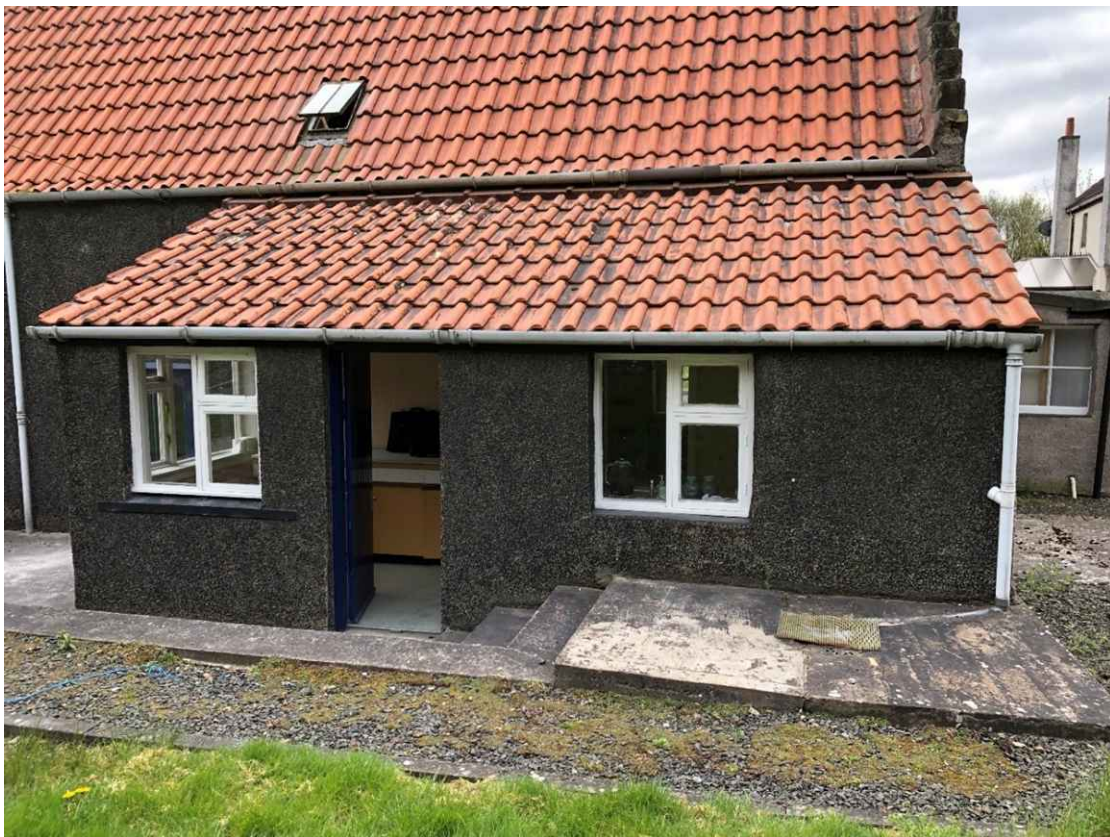
Victorian kitchen addition to the rear of the cottage with mono pitched roof tucked under the eave line. A conservation skylight is also visible on the cottage's roofline. It is clear that this extension also received a new roof in the 1980's when the dark grey cement render was applied.
