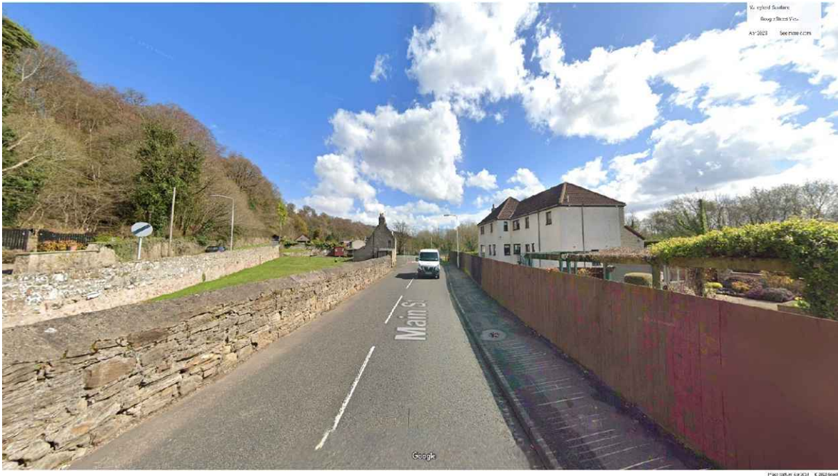
View east towards Westend Cottage showing #6 Veere Park dominating the visual interpretation of Westend Cottage. The two-storey building has an imposing and direct impact on the visual amenity of the listed building without recognising the listing status. This building has a huge impact on the interpretation of Westend Cottage in terms of scale and mass. The rise of the bank to the north and the tree line also provides a large scale backdrop to Westend Cottage all of which are considerations in the context of scale and mass for any development of the site.
