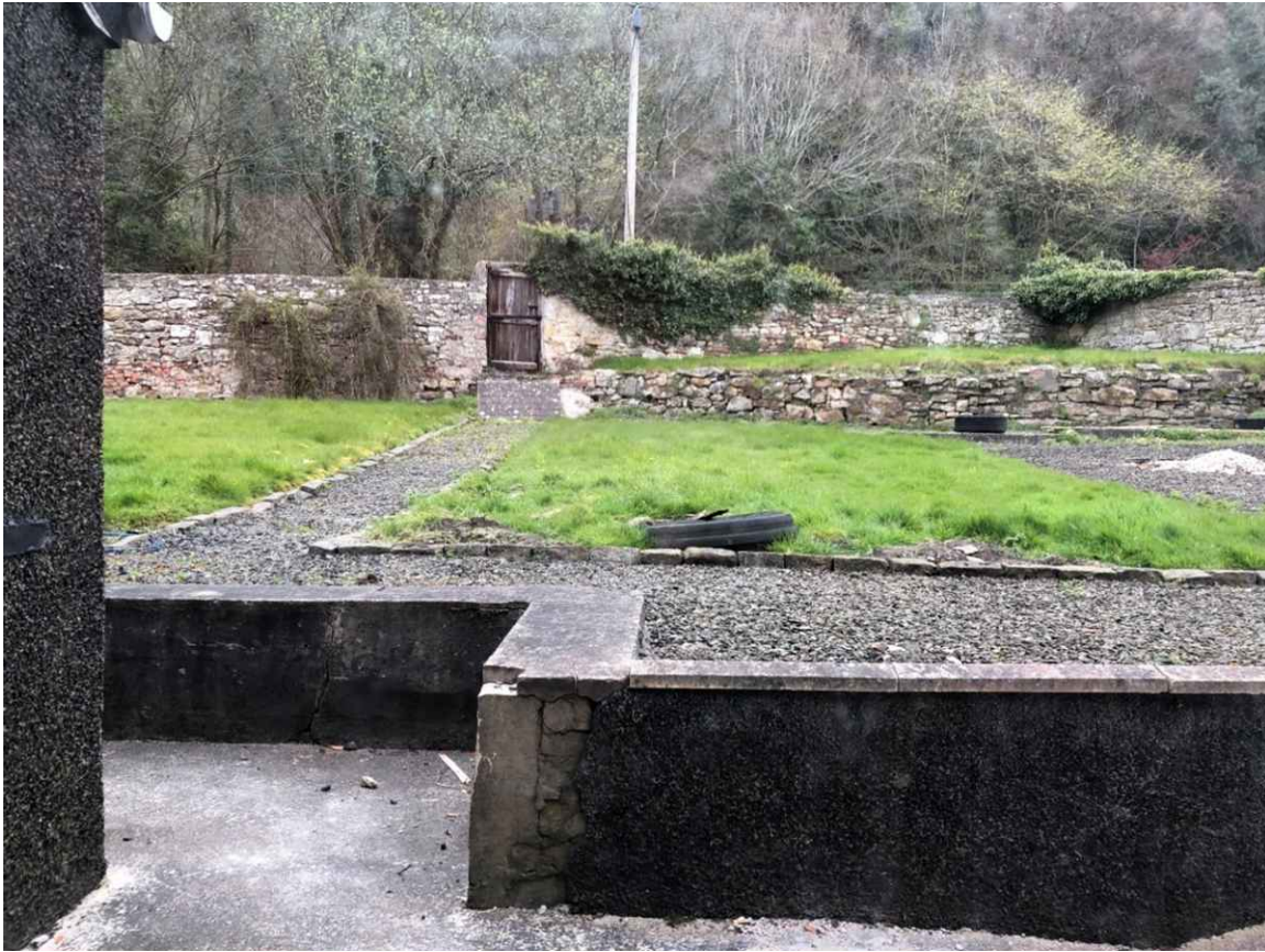
Figure 7: View looking north from the listed building showing the extent of the site's change in levels. Low Causeway Road is beyond the north boundary wall with the pavement being set down by 1.6 – 1.8m. The proposed north extension is to be located in this spot.
