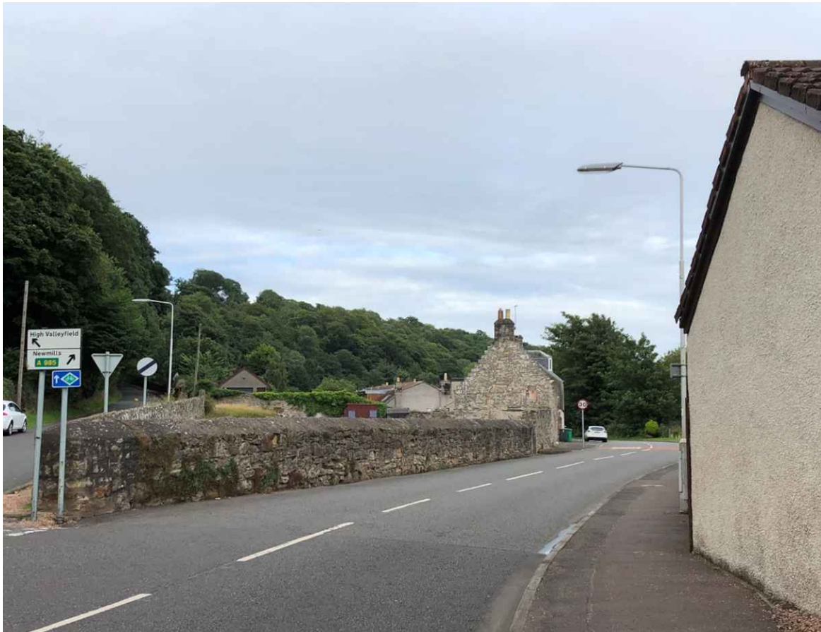
Figure 8: View into the property from the west showing the boundary wall and Low Causeway Road to the northeast. The boundary wall to the north prevents overlook into the site. The Veere Park development is to the right and as Westend Cottage is gable facing to the road, it blends into the existing landscape.
