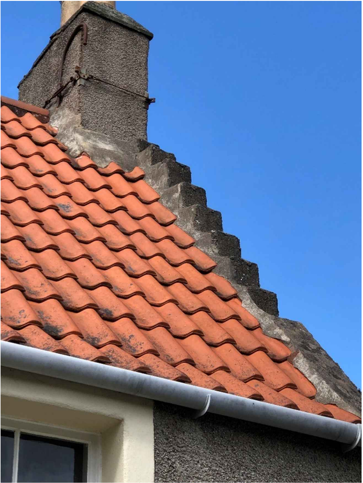
Change in roof line and pitch shown on south side at the east gable where the lower crowstepped stones have been covered in cement to smooth out the pitch
