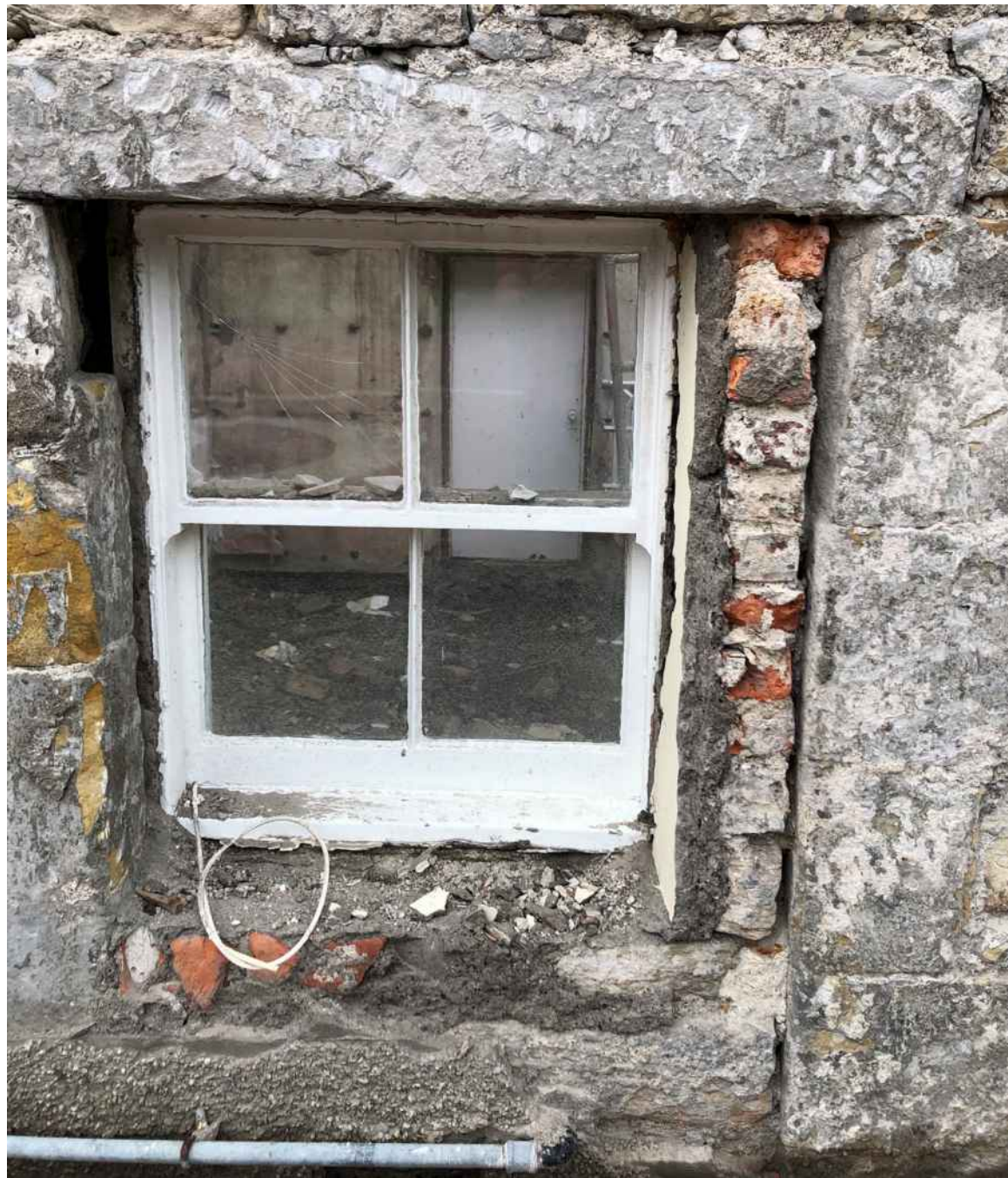
Figure 23 above and 24 below: Image of window with stripped out box for sash and case so that the window fitted the opening. These windows were installed in the mid-20th century and are non-operational. Removal of the render as shown dates window installation to that of the time of render. The windows no longer fit the cottage with the cement removed and the windows returned to their original sizes.
