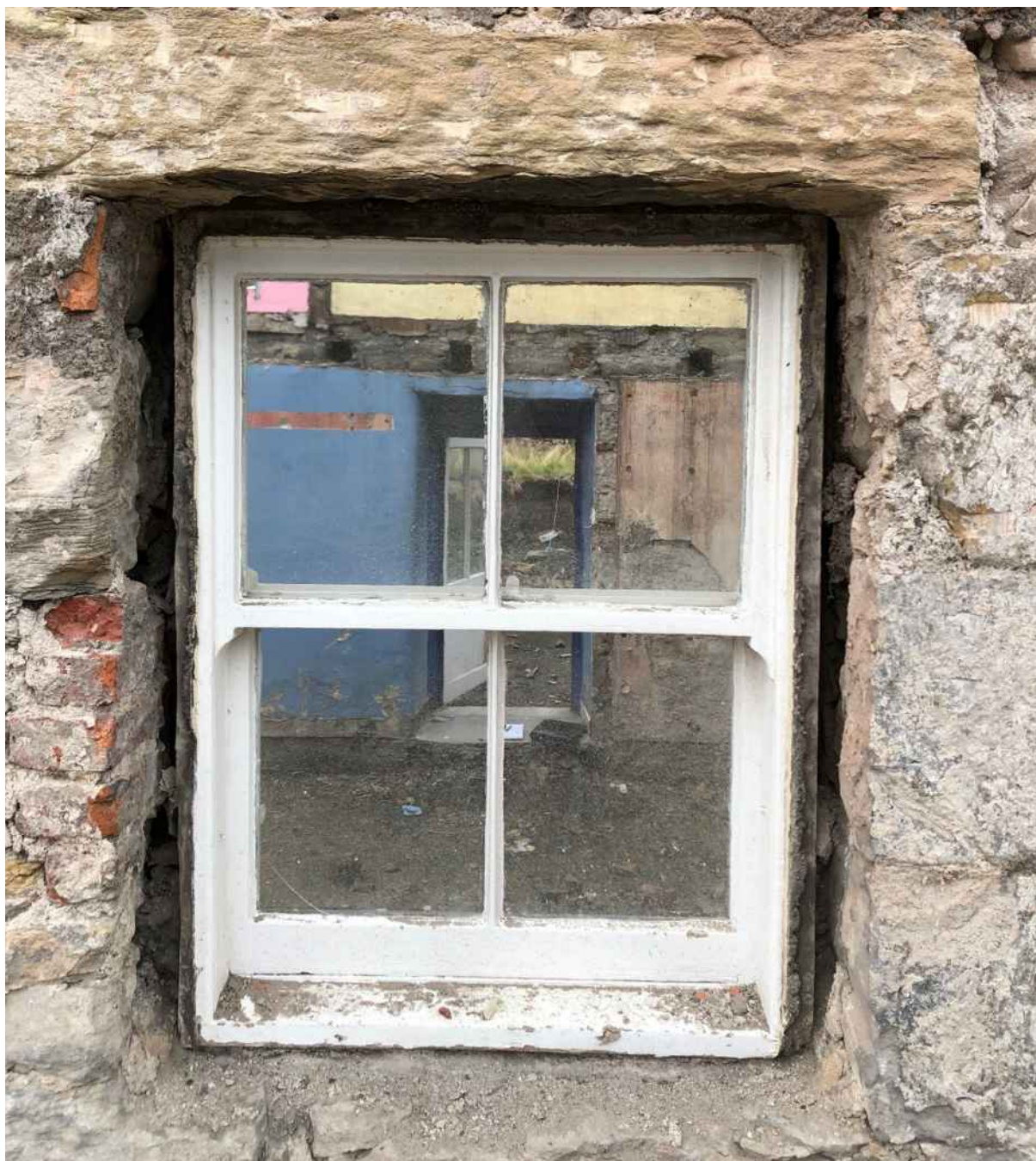
Figure 23 above and 24 below: Image of window with stripped out box for sash and case so that the window fitted the opening. These windows were installed in the mid-20th century and are non-operational. Removal of the render as shown dates window installation to that of the time of render. The windows no longer fit the cottage with the cement removed and the windows returned to their original sizes.
