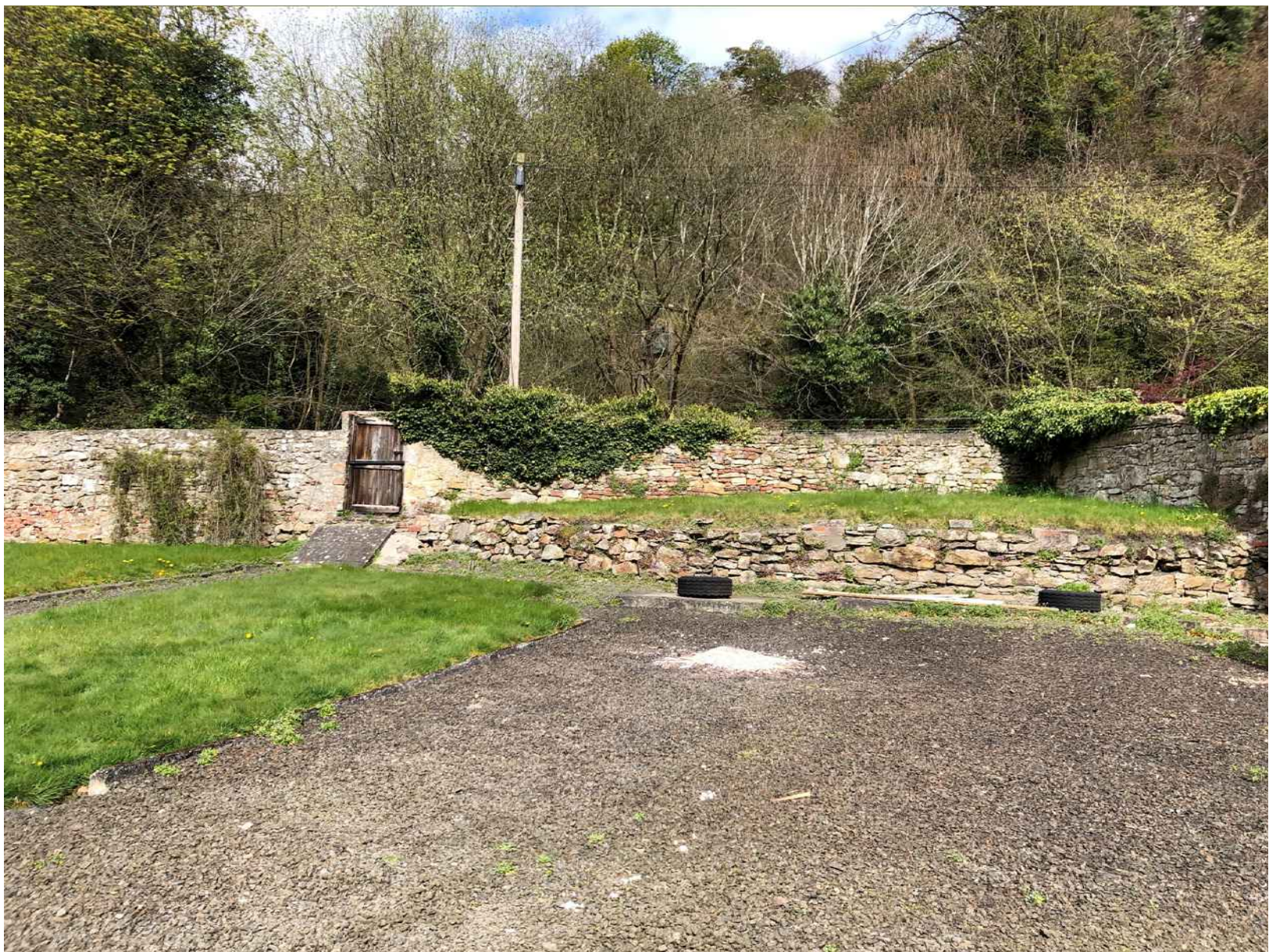
Figure 4: View of northern boundary wall and change in height of rear garden. The rear extension will sit down into the site by approximately 1.5m where the grass section is shown to the left of this photograph.
