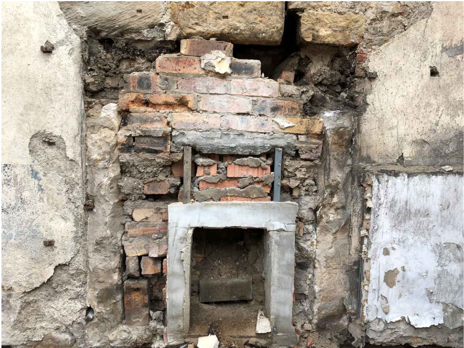
Figure 29: Image of uncovered original stone fireplace frame with missing lintel and the impact of the imposition of the Victorian fire chamber. This will be opened with a new stone lintel installed.
