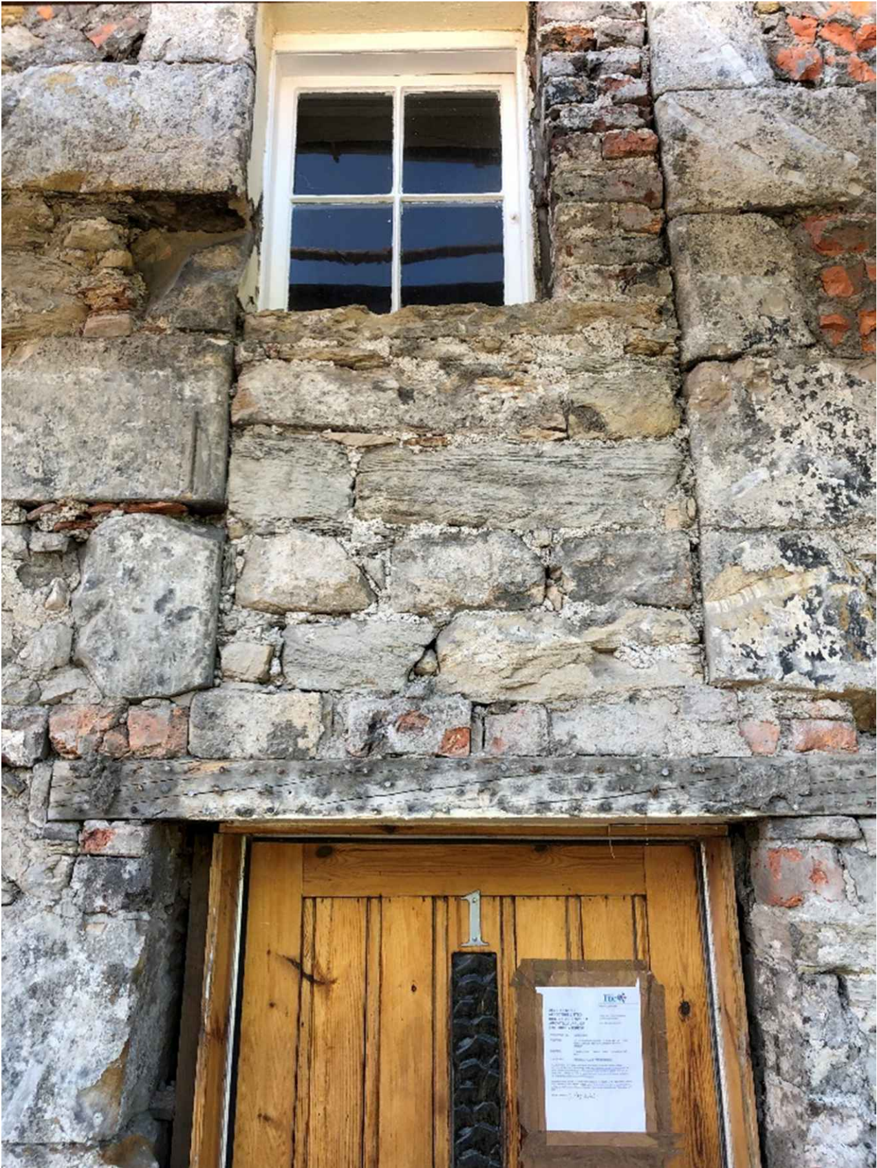
Figure 1: Quoined returns at the front door that show the building was once two distinct buildings. The quoins run down to grade
