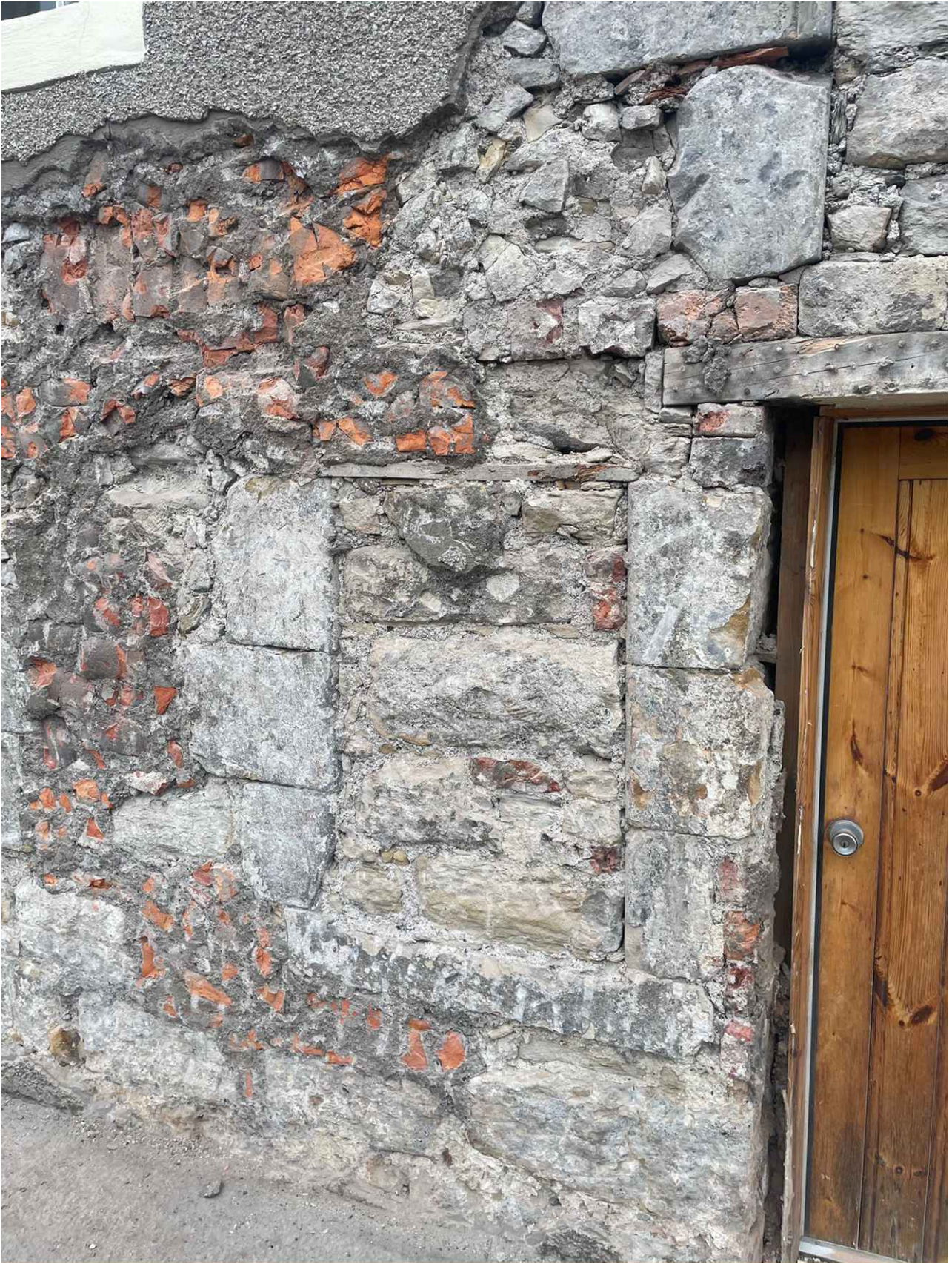
Original window filled in with sandstone to the west of the front door. Brick and cement infill to fill in gaps in the wall for the cement render applied in the 1960's.
