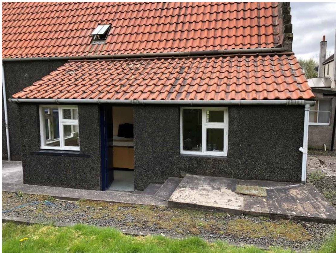
Victorian kitchen addition to the rear of the cottage with mono pitched roof tucked under the eave line. A conservation skylight is also visible on the cottage's roofline. It is clear that this extension also received a new roof in the 1980's when the dark grey cement render was applied.
