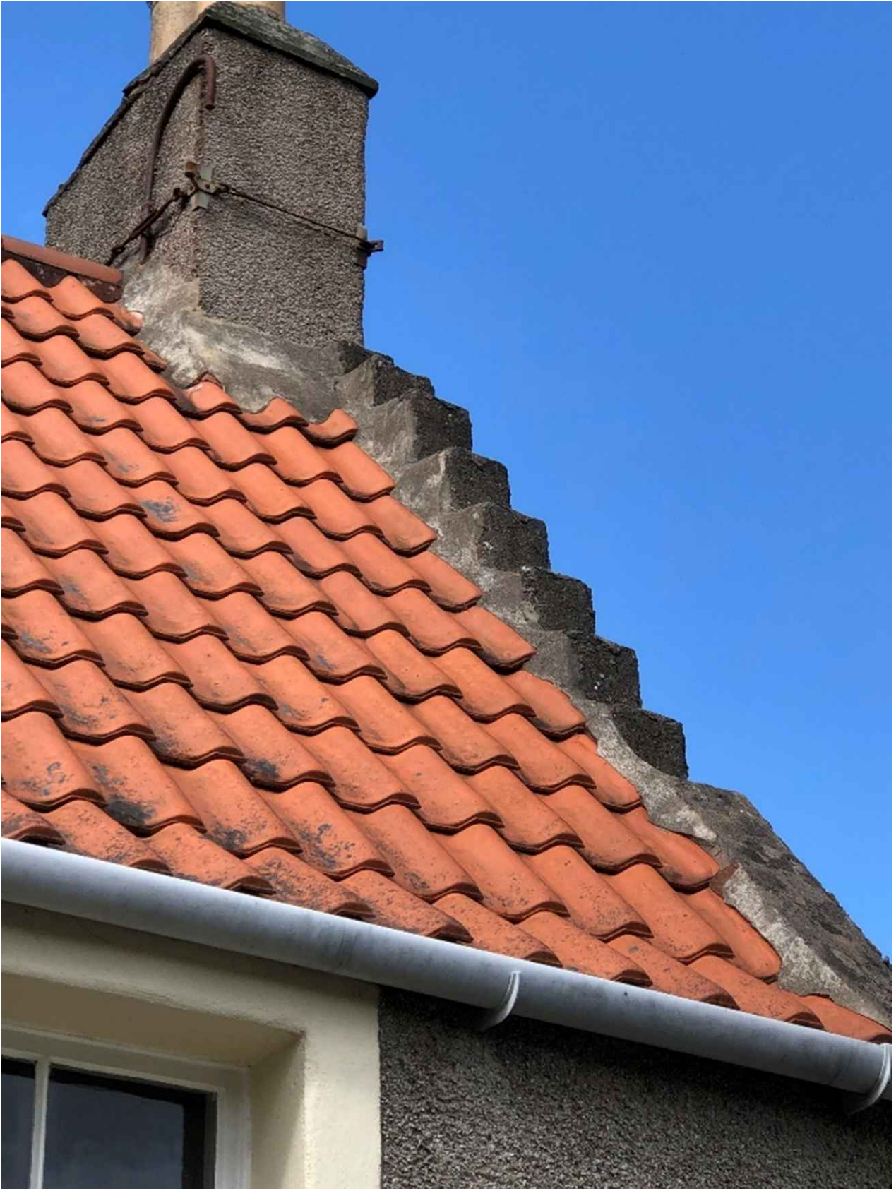
Change in roof line and pitch shown on south side at the east gable where the lower crowstepped stones have been covered in cement to smooth out the pitch
