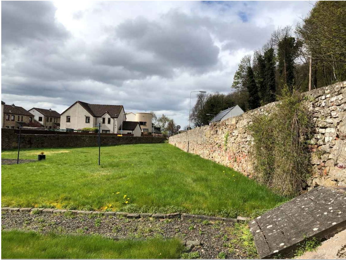
View of the property from the north boundary wall looking west
