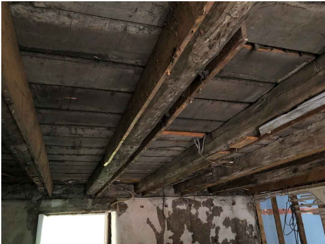
Sistered floor joists using 1" material. The floor joists were full of dry rot and had no load bearing capacity left. They had been sistered by timbers inadequate for their structural use and the resultant impact was a failure in structural integrity.
