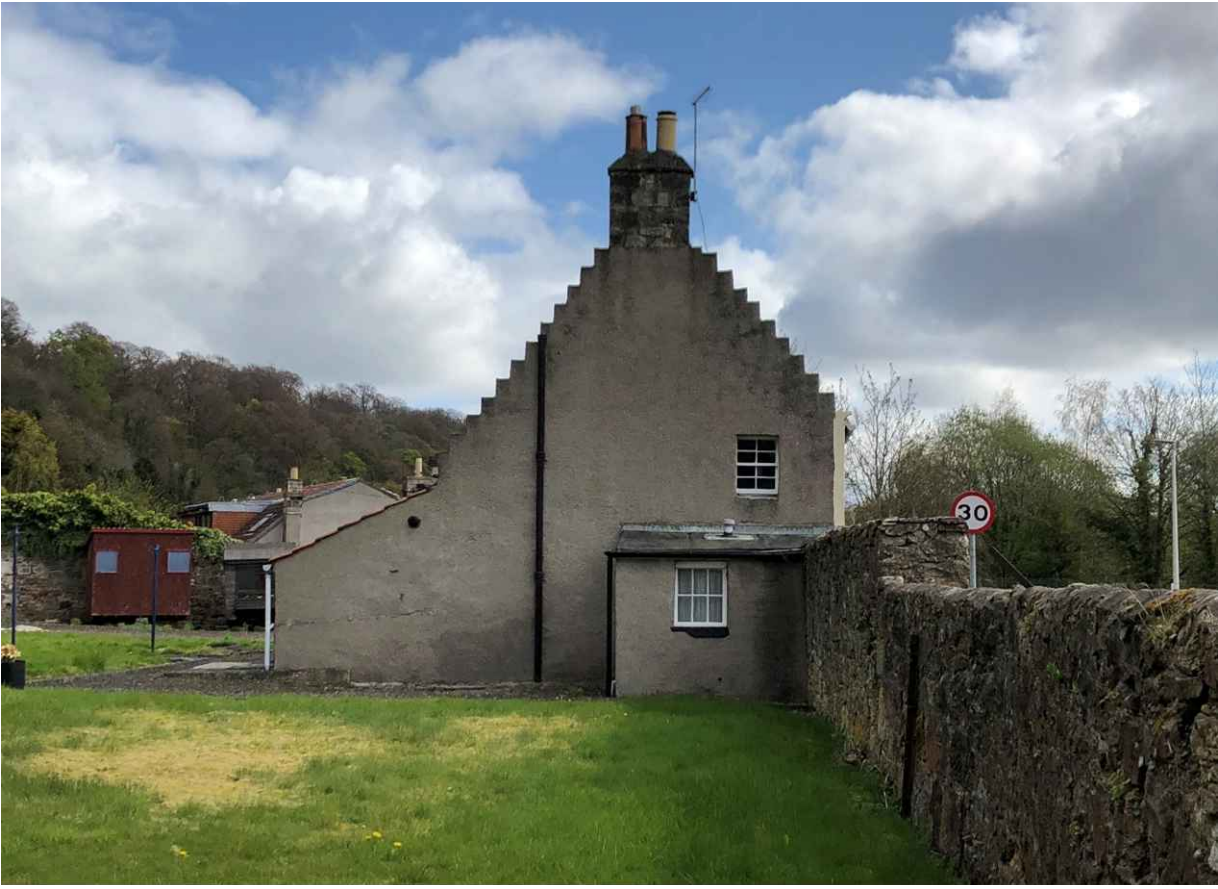
View of the property looking east
