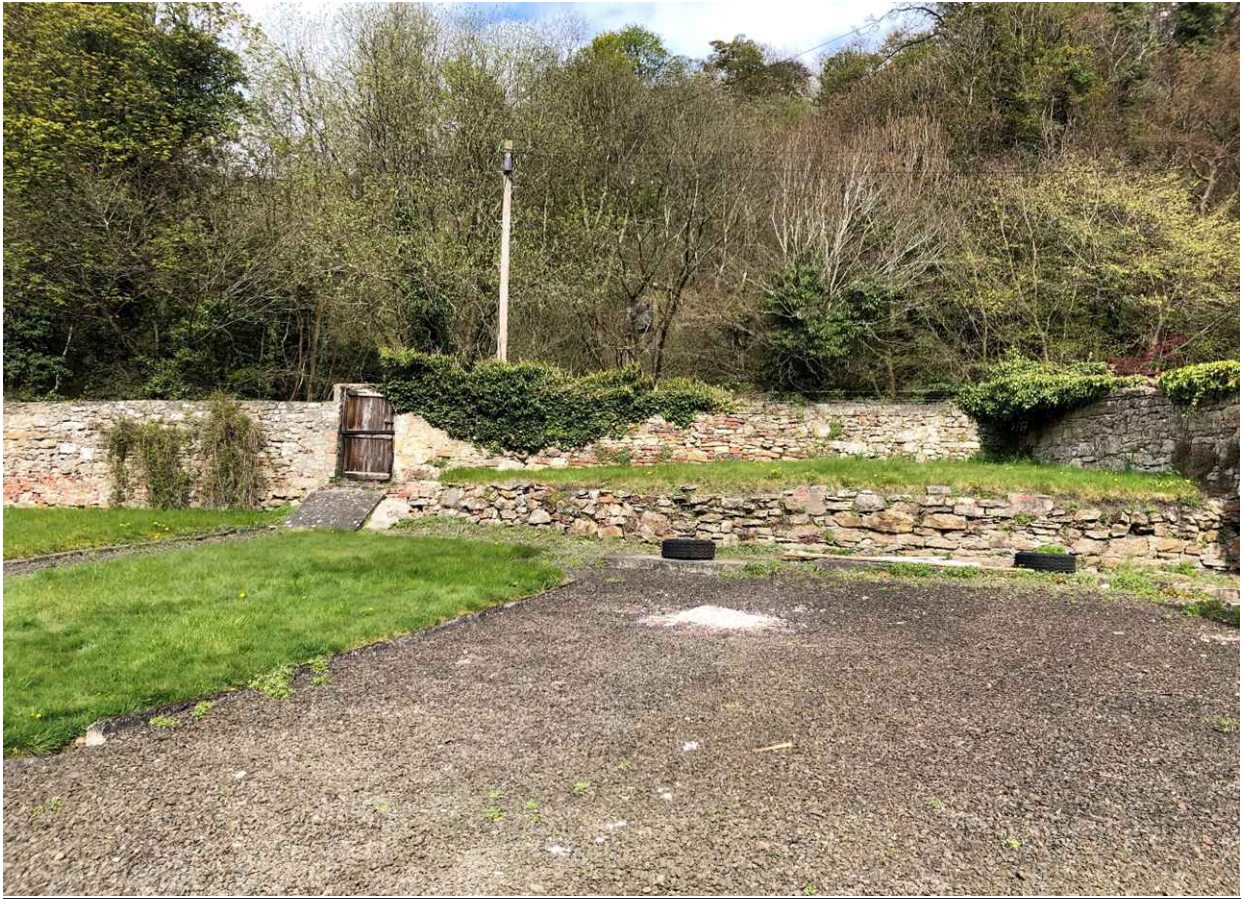
View of the property looking to the north boundary wall showing change in elevation of the property to the north boundary wall
