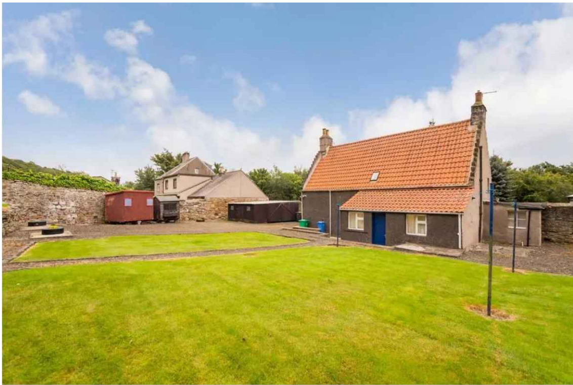
View of the north of Westend Cottage showing the location of the proposed extension
