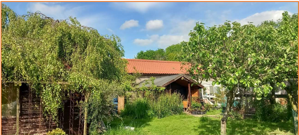
Photo 1 – showing the building and garden area for the building
