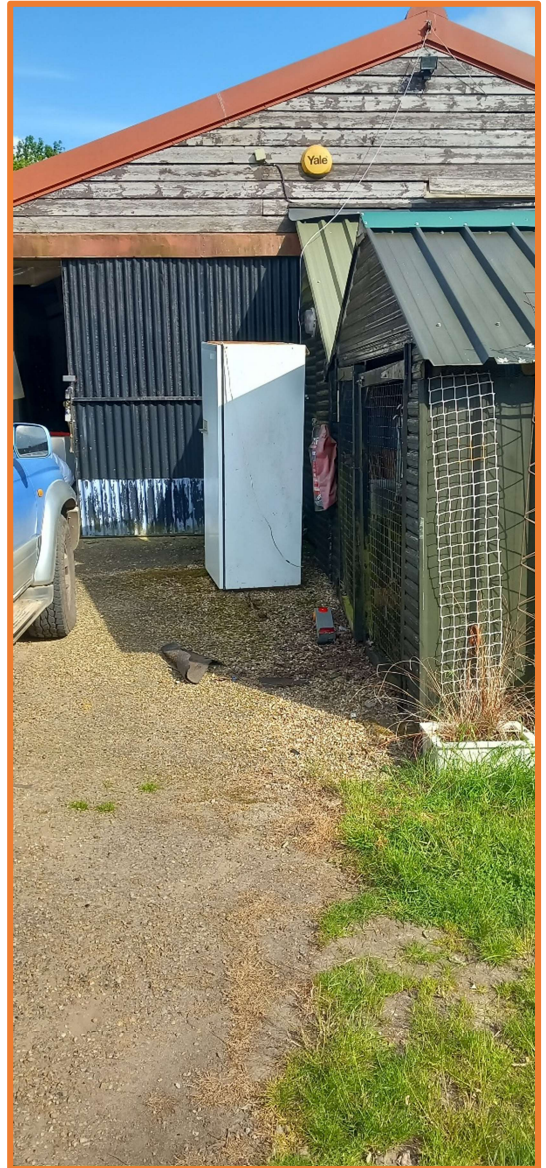
Photo 2 – Showing existing entrance to building
