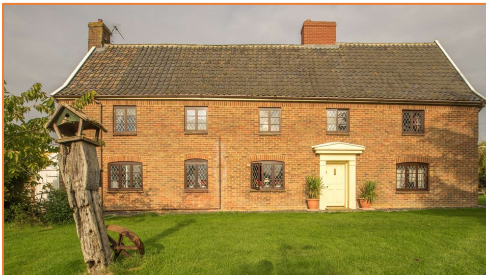
Figure 2: Photograph of the front elevation of Row Farmhouse
