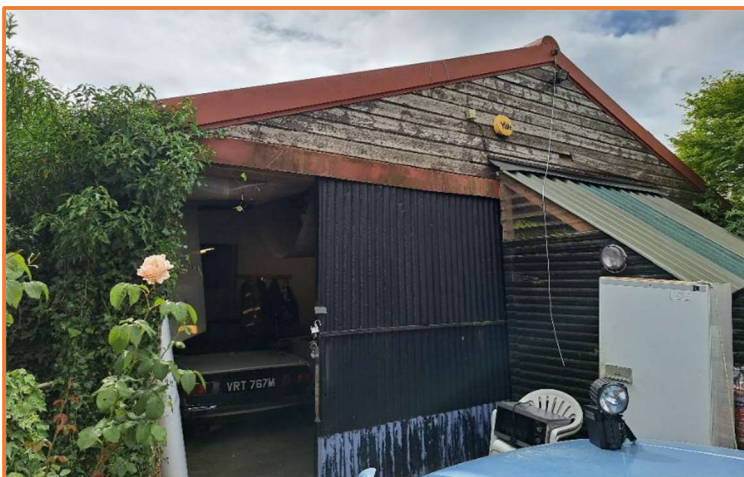
Figure 4: Photograph of existing barn elevation
