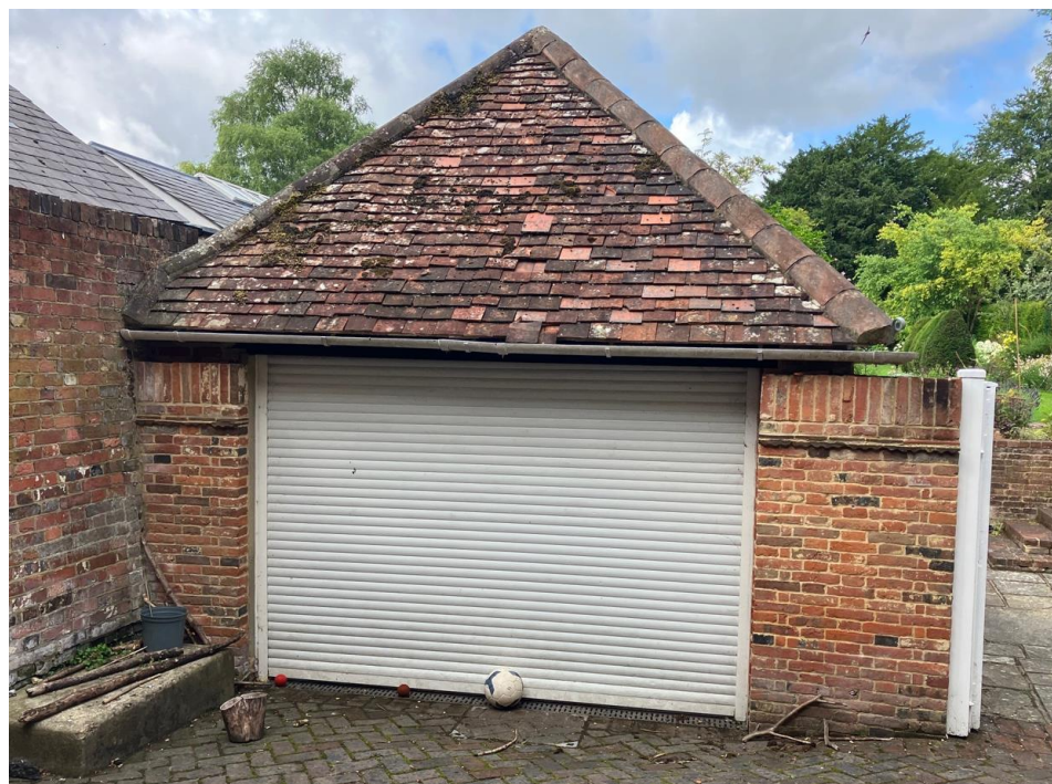
Figure 5 – Garage door photograph, in context
