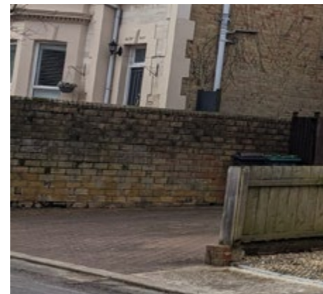
permeable paving and brick boundary wall
