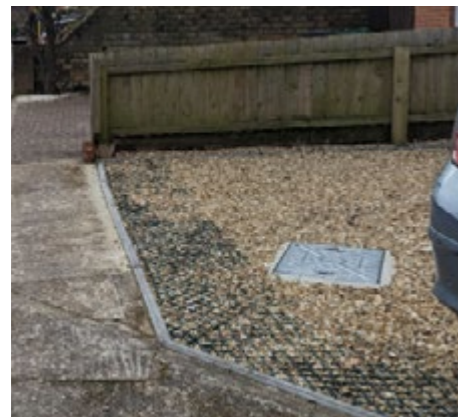
gravel and timber fencing
