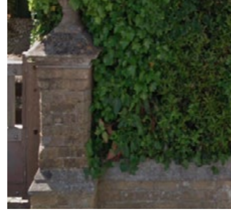
Buff brick on the site boundary
