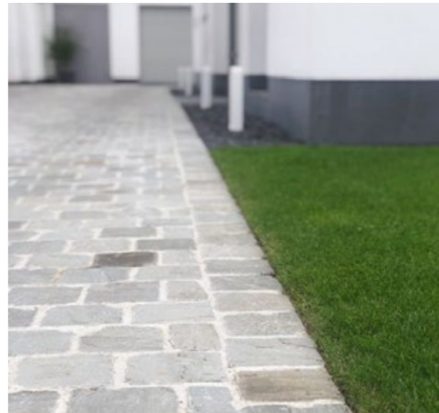
Permeable Block Paving on driveway.
