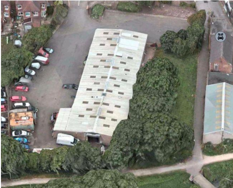
Aerial view of the site.
