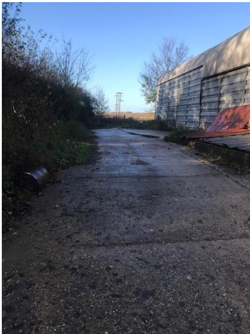
EXSITING ACCESS TO FRONT OF BUILDING
