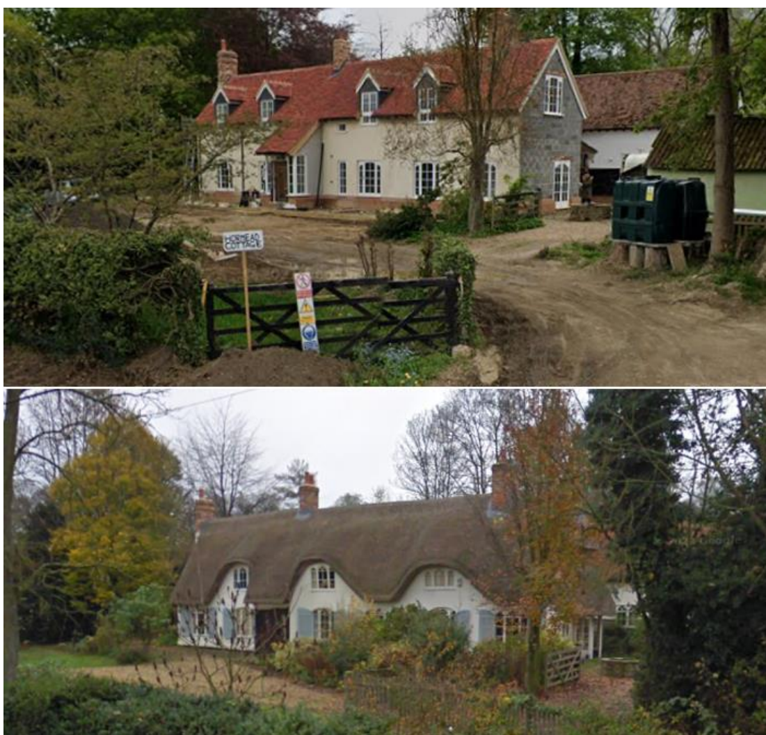
Fig.23: Hormead Cottage in 2023 (top) and in 2009 (bottom). As a result of fire destruction in 2016, the property was rebuilt in 2018, retaining limited ground floor fabric and chimneys but a different first floor layout and roof type. Source: Google Street View.
