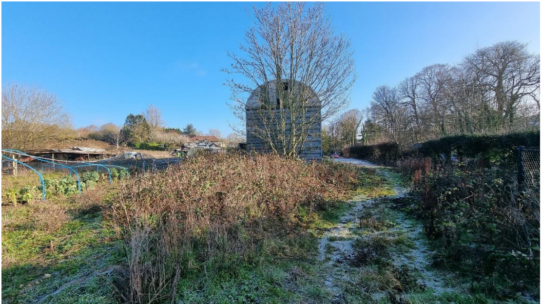
Fig.8: The west elevation of the grainstore with road to the right.
