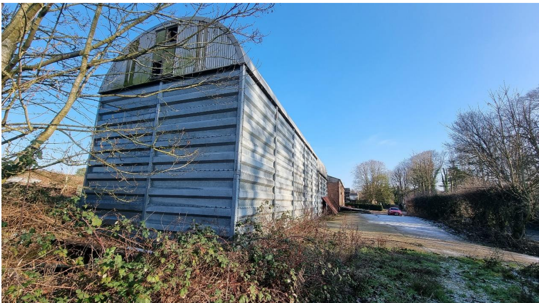
Fig.4: The metal construction store at the western half of the site.
