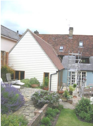
Site Photo 2: Rear Elevation
