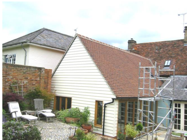
Site Photo 3: Rear Elevation
