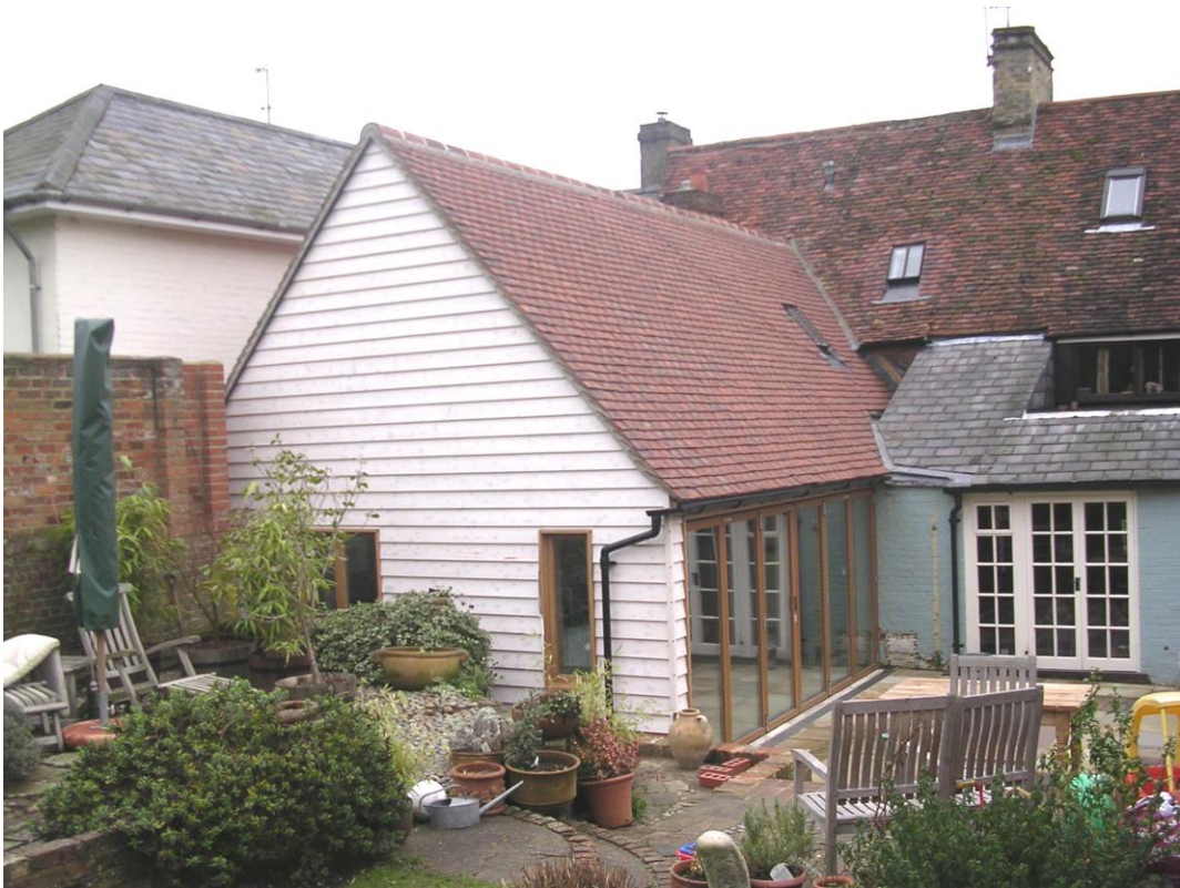
Site Photo 1: Rear Elevation of Crown House with 2004 extension in Foreground
