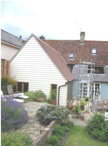
Site Photo 3 : Rear Elevation
