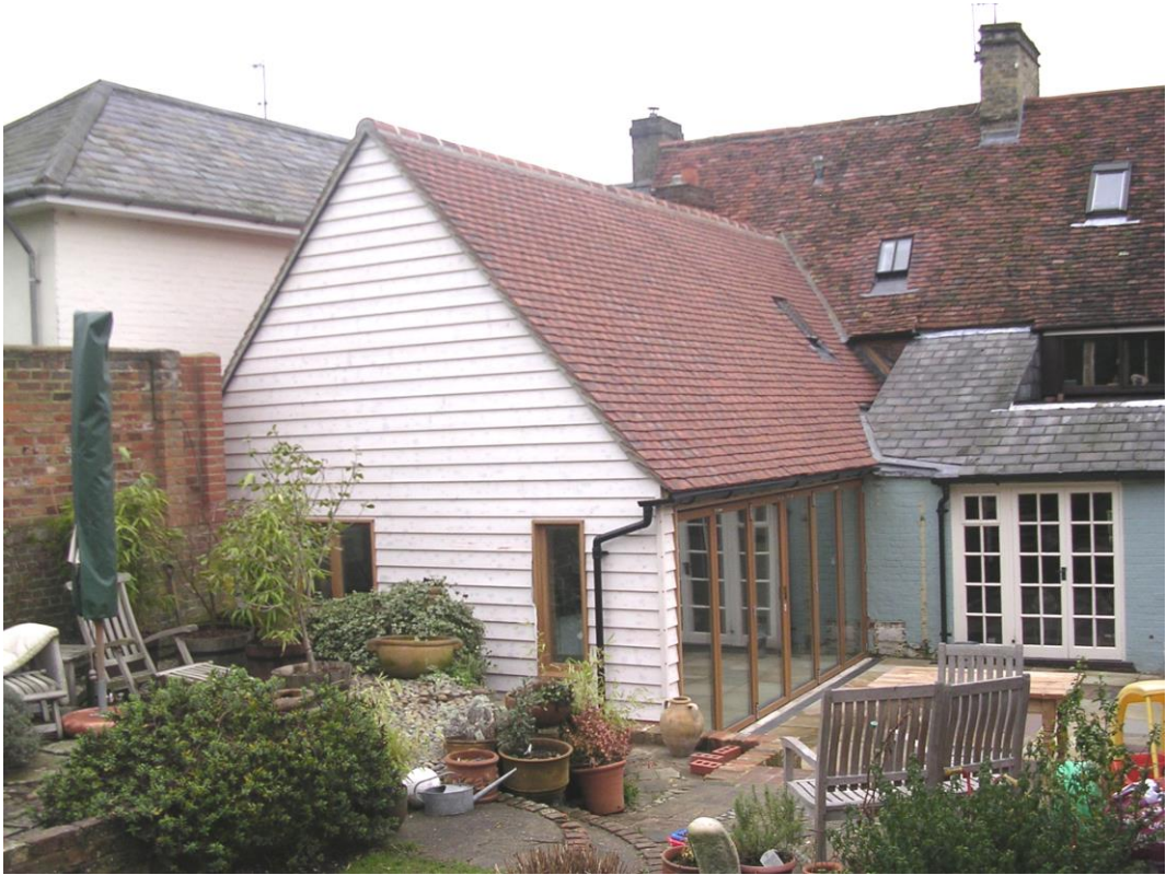
Site Photo 2 : Rear Elevation
