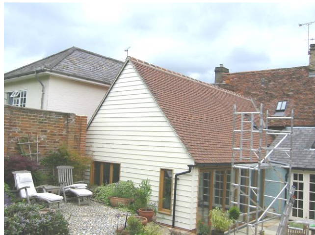
Site Photo 4 : Rear Elevation
