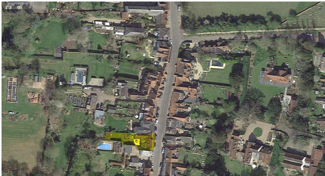
Aerial View of site (Courtesy of Google Maps) (existing highlighted)
