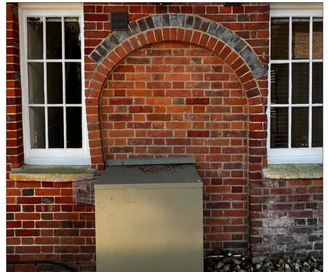
Figure 2: former opening to stables now bricked up
