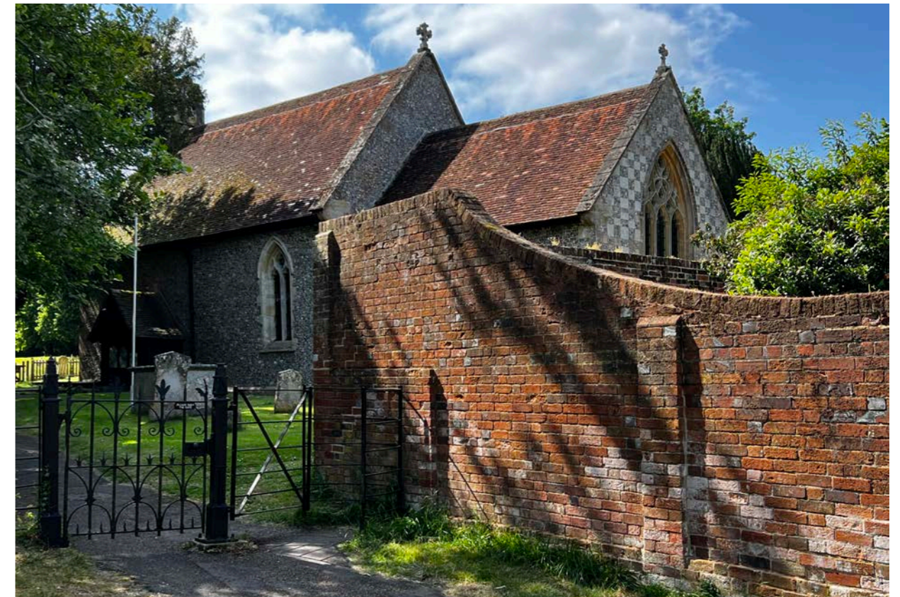
Figure 7: Holy Trinity Church with flint checkerboard construction and high brick boundary wall of the Old Rectory
