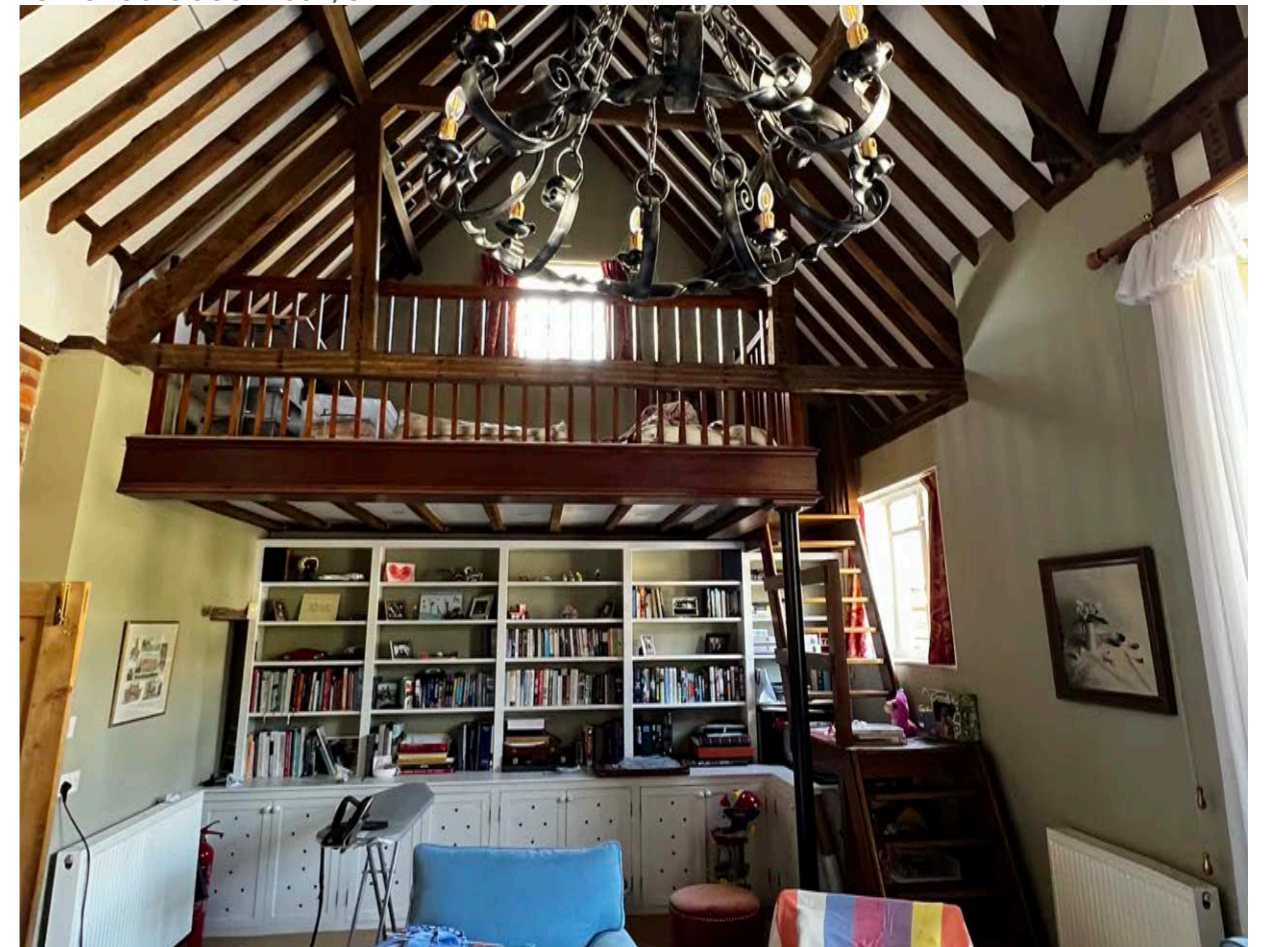
Figure 6: former library converted to sitting room with gallery and stairs added
