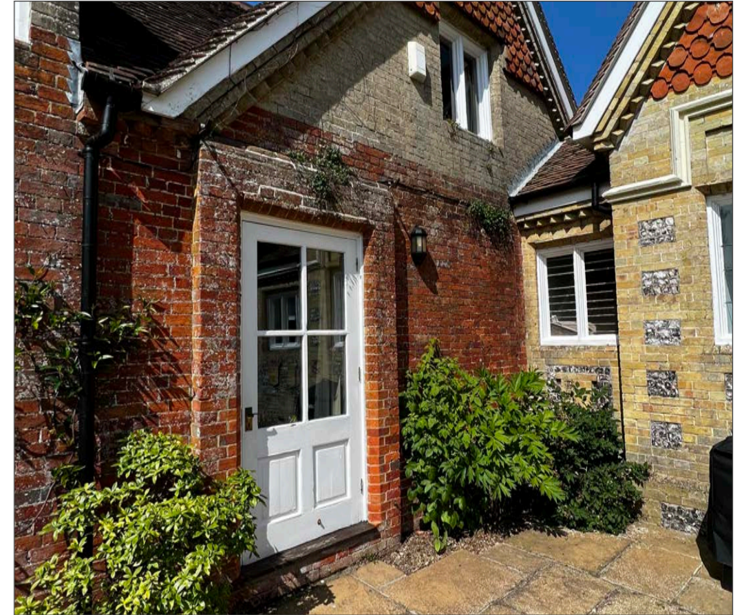
Figure 1: door from existing kitchen
