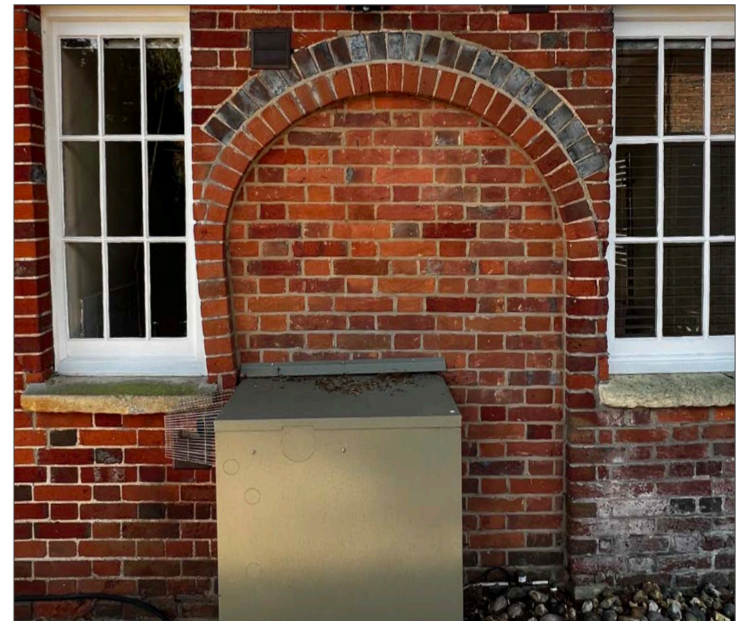
Figure 4: former opening to stables now bricked up to be re-opened
