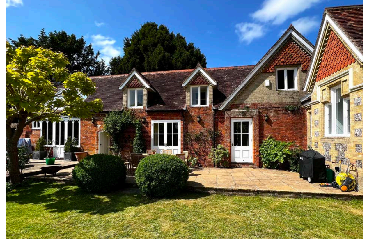
Figure 3: new dormers built to first floor over kitchen and breakfast room around 1993 and proposal to place window to right of the single door to create additional natural light
