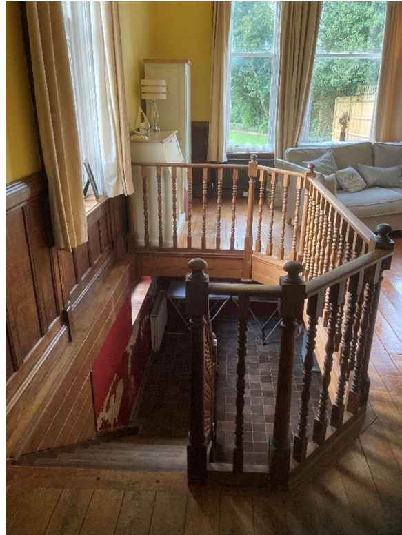
Fig.9 – Photograph (2) showing the staircase in the living room leading down to the basement
