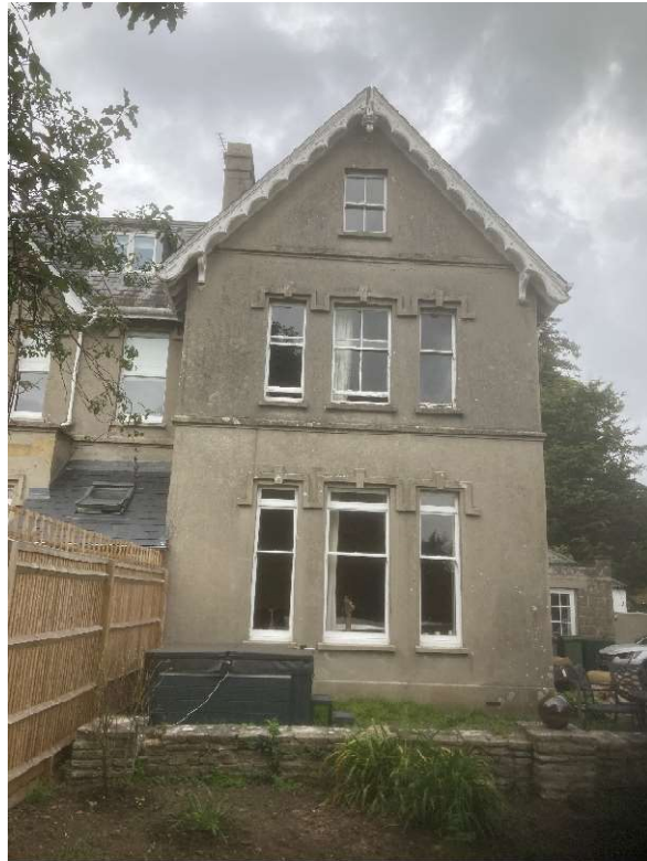
Fig.1 – Photograph showing the south-west elevation of 8 Hall Court
