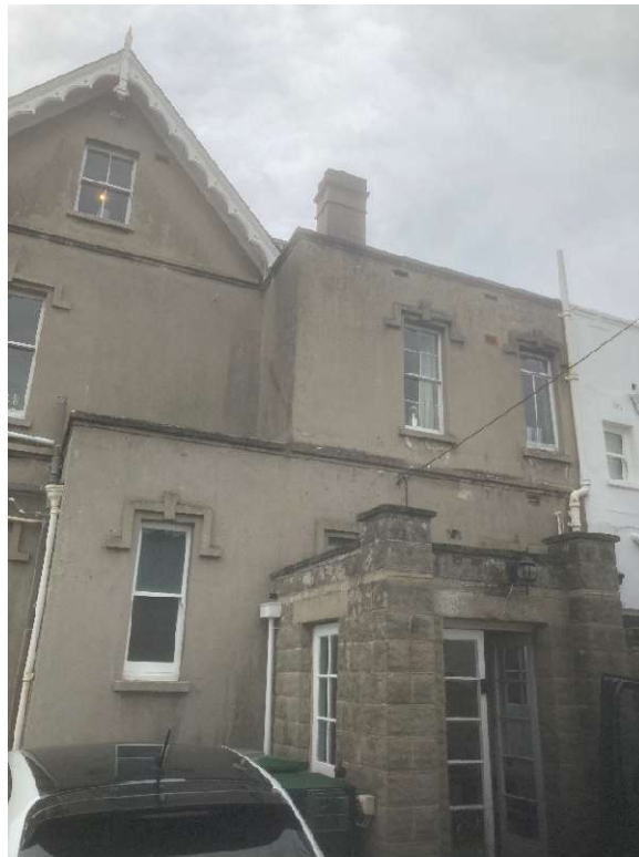
Fig.4 – Photograph showing the south-east elevation of 8 Hall Court
