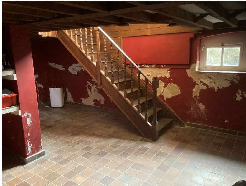
Fig.11 – Photograph taken in the basement looking towards the staircase and window
