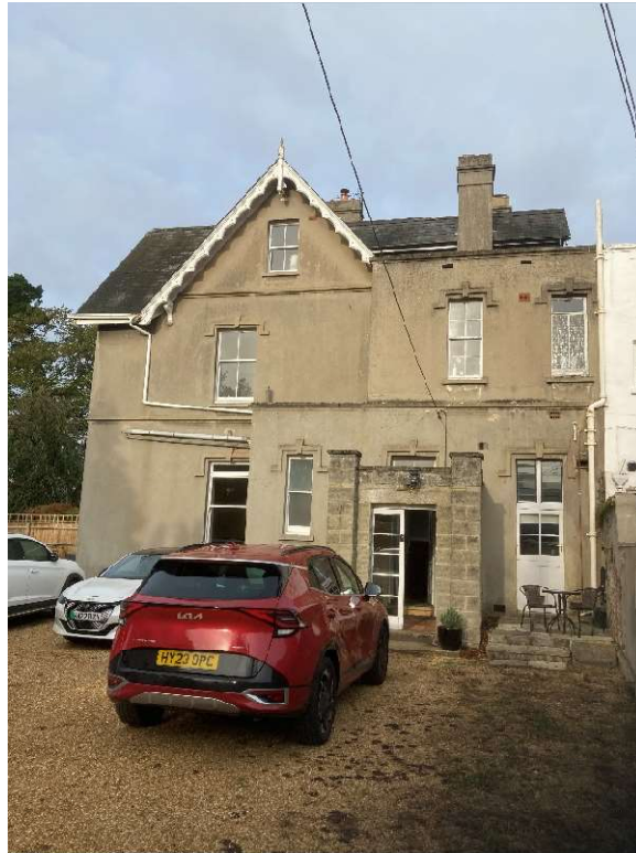
Fig.3 – Photograph showing the south-east elevation of 8 Hall Court with the porch added as a later addition to the property
