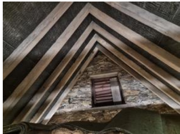
Figure 17: view of loft area, looking east (vents blocked up on outside).
