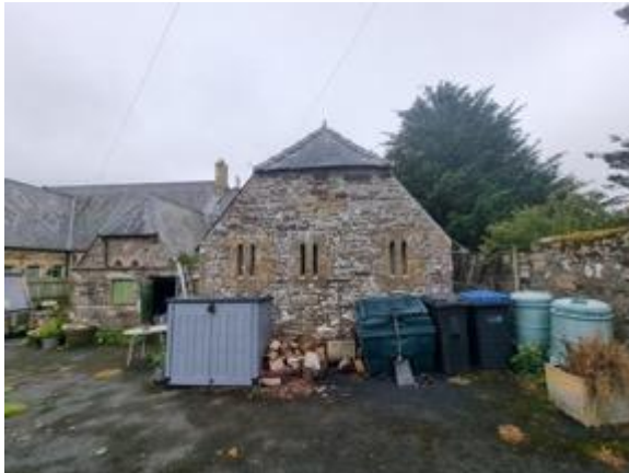
Figure 10: B1 - rear/W elevation.
