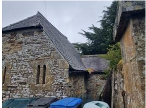
Figure 11: B1 -SW elevation showing rear of coal shed attached.
