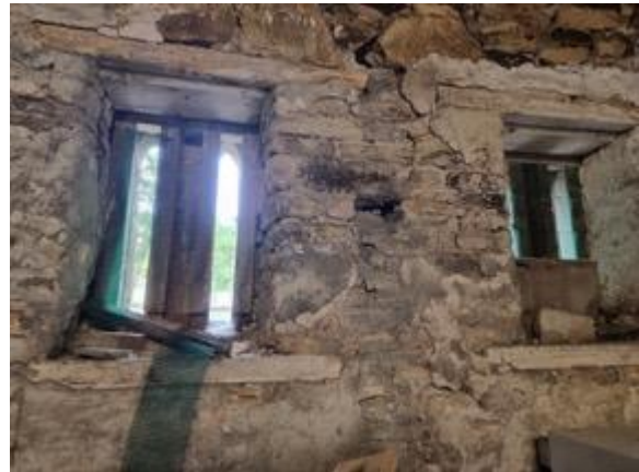
Figure 19: inside vents on west wall of building
