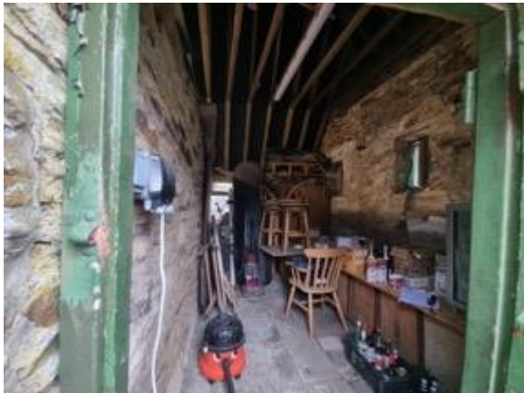
Figure 18: Inside of rear/west of building
