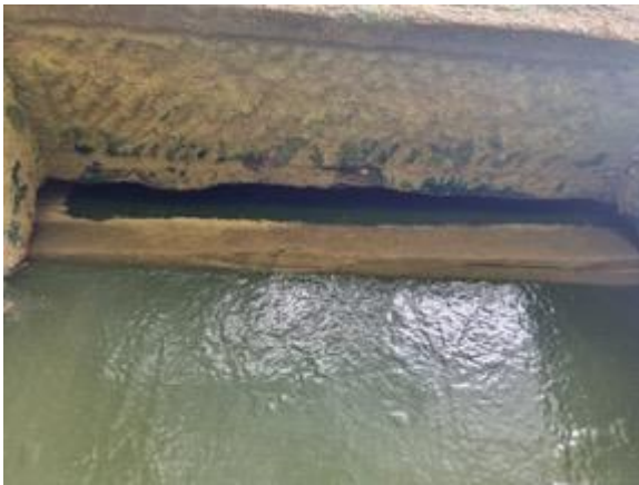
Figure 24: gaps in lintel above windows
