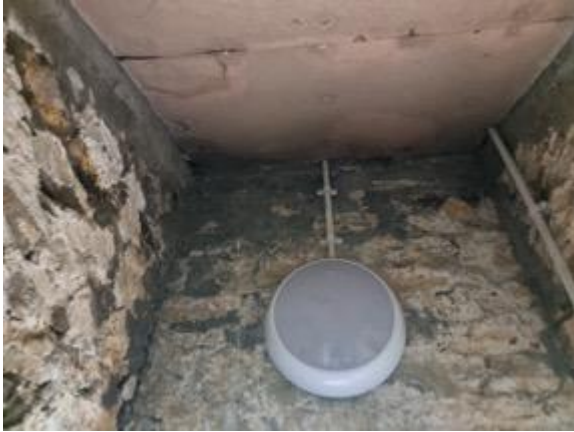
Figure 26: inside of coal shed.
