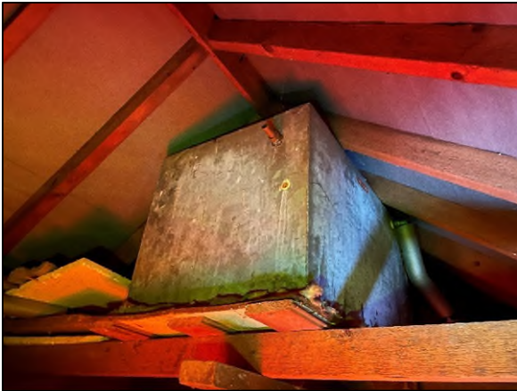
Plate 7: view of loft void 2 in B1.
