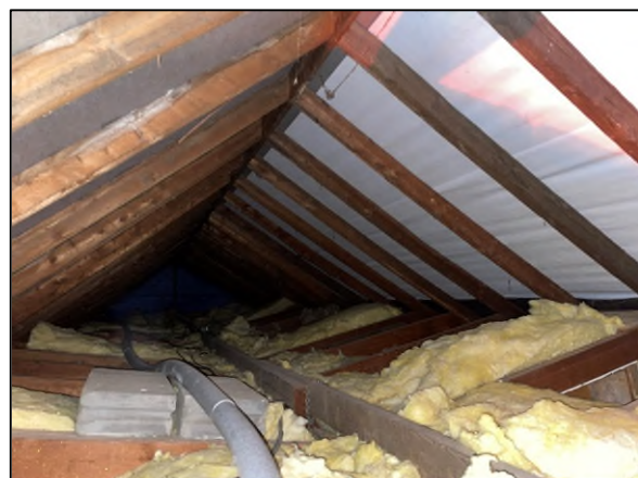
Plate 6: view of loft void 1 in B1.
