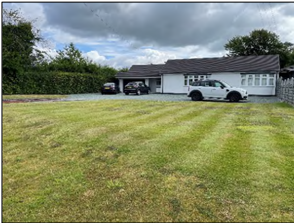
Plate 1: typical view of the site. Photograph looking east.
