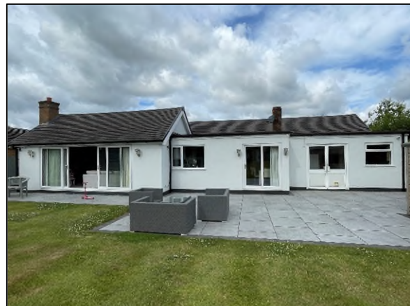
Plate 4: view of The Owls Nest (B1). Photograph looking west.
