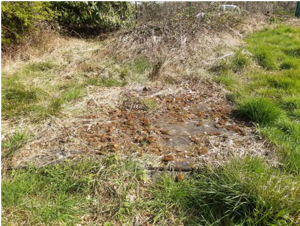
Fig. 29: Concrete Slab at Top of Terrace Looking North-West
