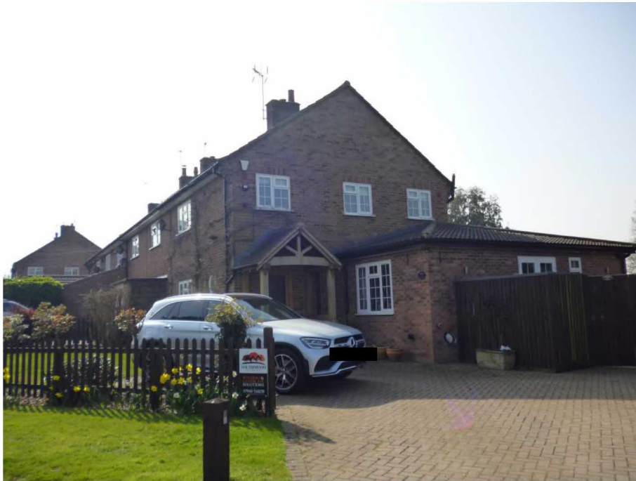
Willow Row – looking at the side(northeast) elevation to No. 14
