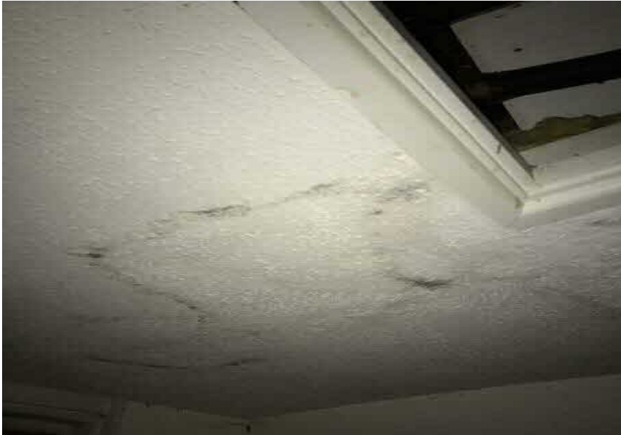
Sample 01 – Textured coating – Chrysotile (white asbestos).
