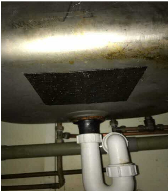
Sample 06 – Acoustic sink pad – No asbestos detected.
