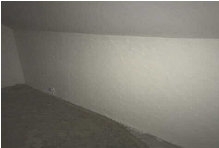
Sample 02 – Textured coating – Chrysotile (white asbestos).
