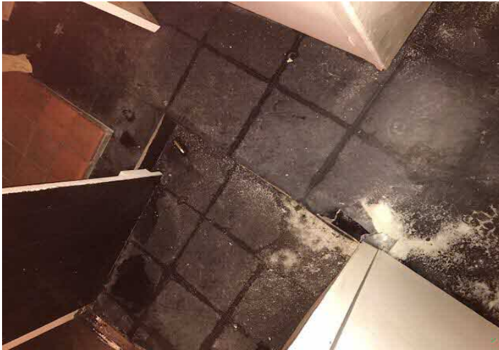
Sample 07 – Floor tiles – No asbestos detected.
