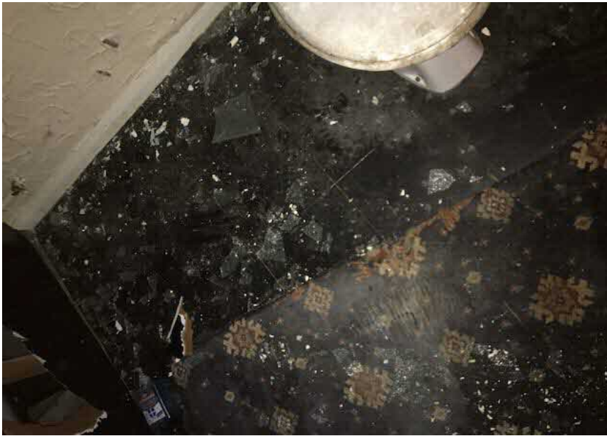
Sample 05 – Floor tiles – No asbestos detected.
