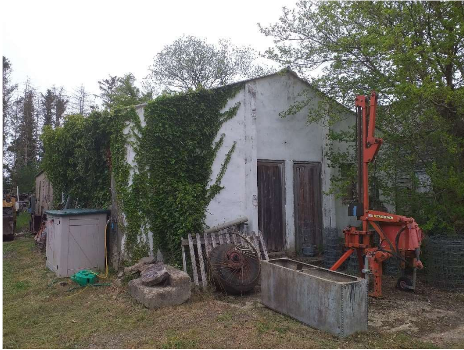
Workshop building southern elevation
