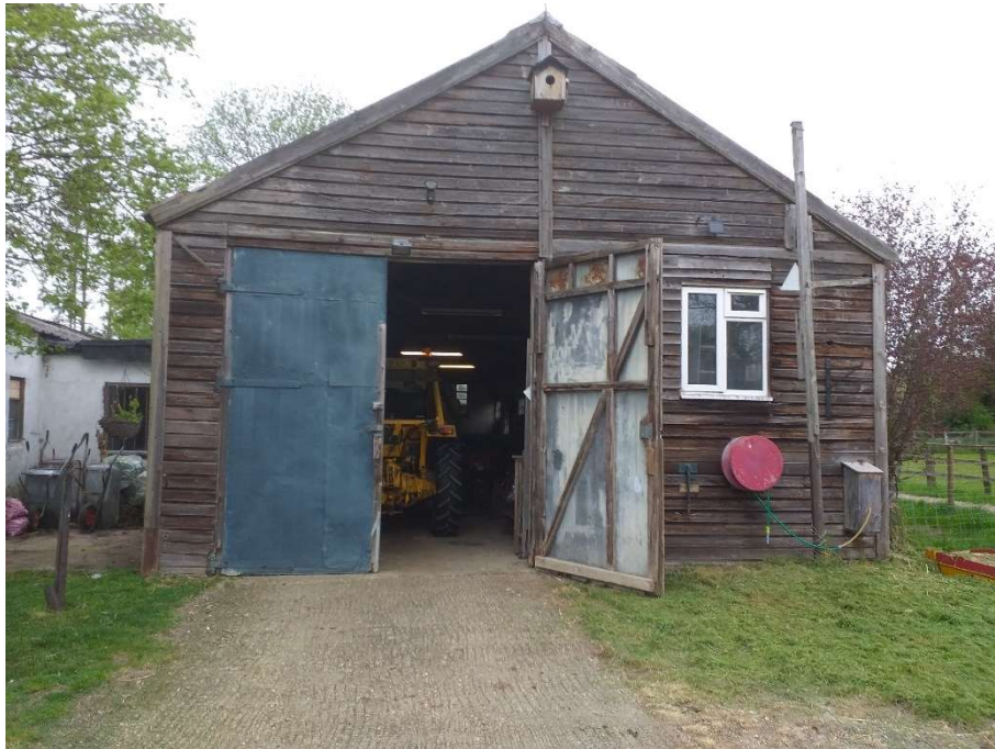
Storage building – southern elevation
