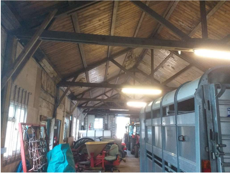
Storage building interior looking south
