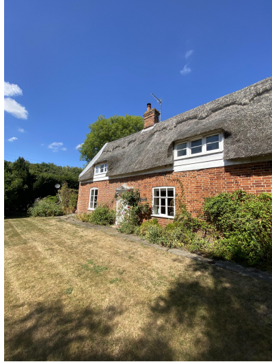
1. South Elevation - Front of Nutmeg cottage
