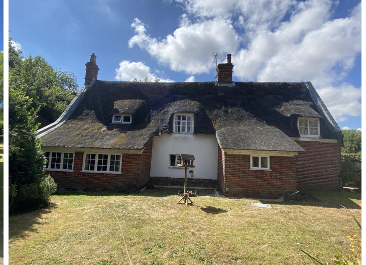
3. North Elevation - Rear of Nutmeg Cottage
