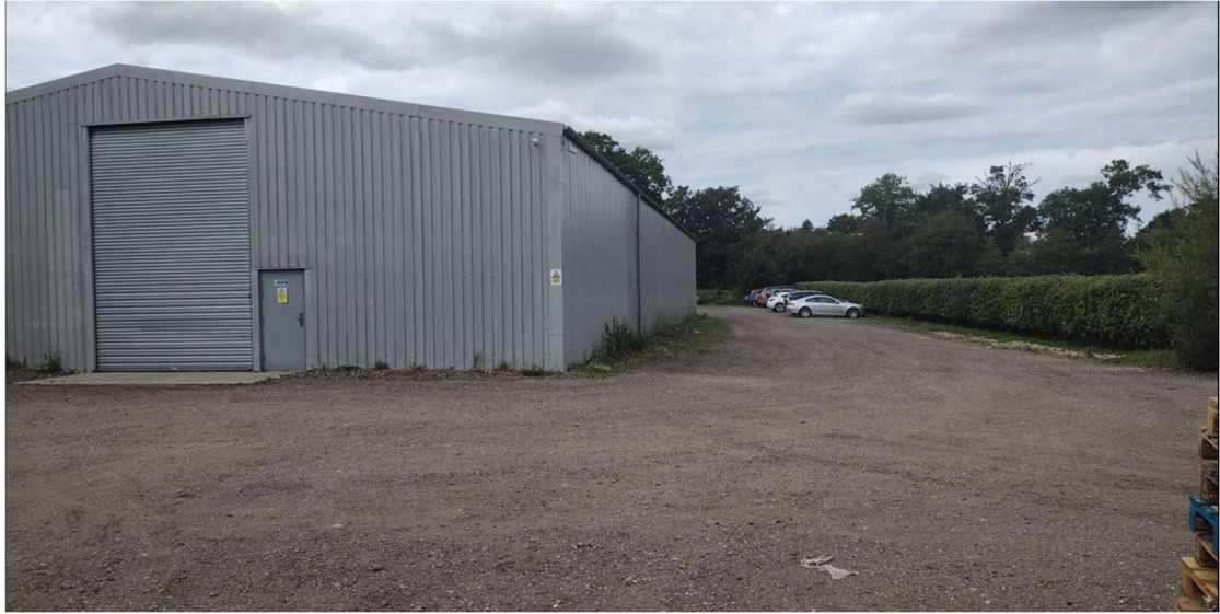
Figure 2 - View from unattended measurement position towards front warehouses
