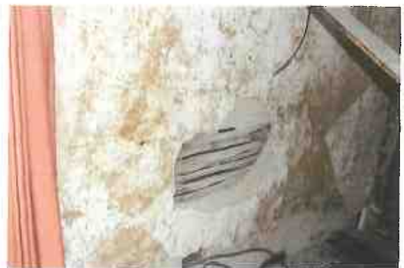
The front wall
