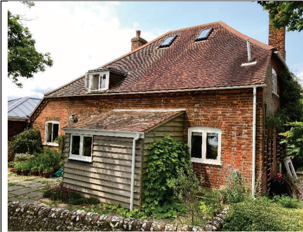
Photograph 1: The eastern elevation of the house
